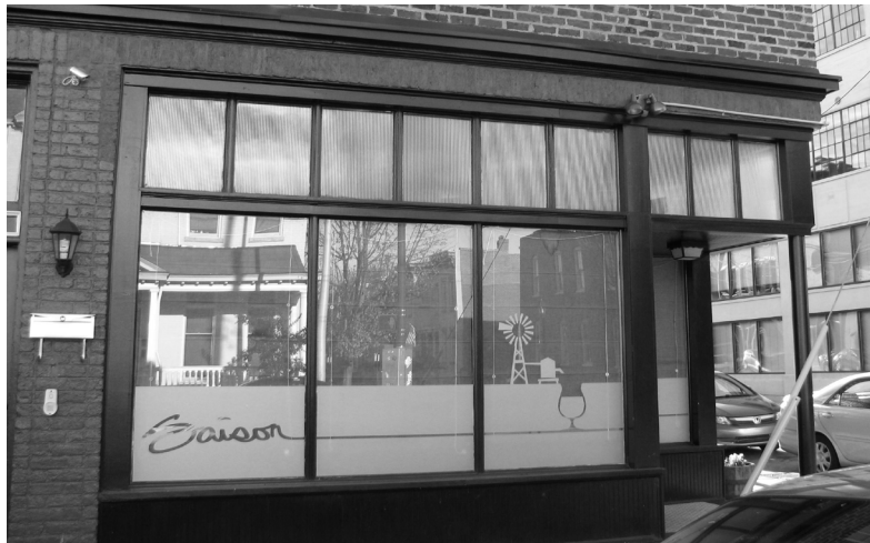
Sunshading and other screens may be necessary for your storefront, but should be removable like these blinds. Windows should not be permanently blocked, covered or reduced in size.
