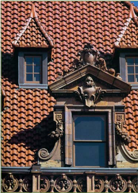
Main Street Station's elaborate architectural details
