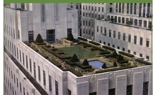
Green roofs, like this one in New York City, can decrease storm water runoff in dense urban areas and provide pleasant views for office workers
