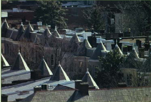
Rooftops on West Avenue mirror and relate to each other creating a rhythm to the street
