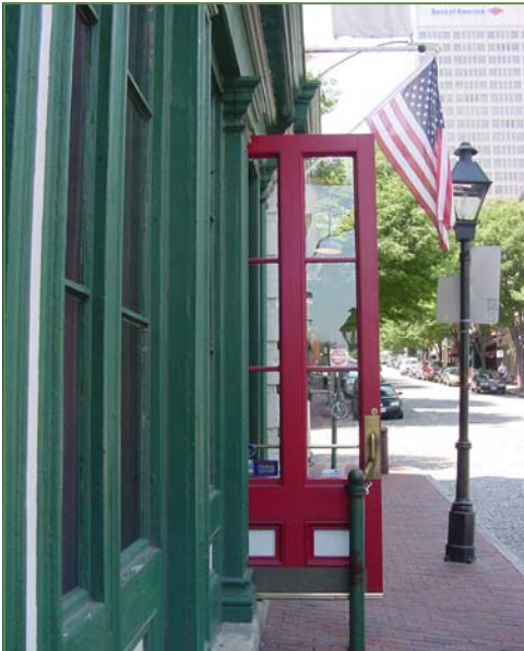
Door swing in Shockoe Slip that could be a hazard for pedestrians
