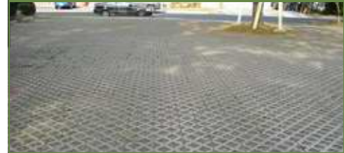
Example of pervious paving as part of a low impact development in Austin, Texas
