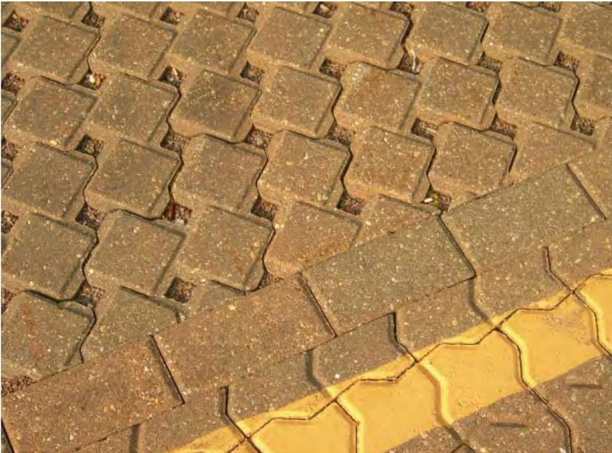
Figure 8.10: Pervious pavers
