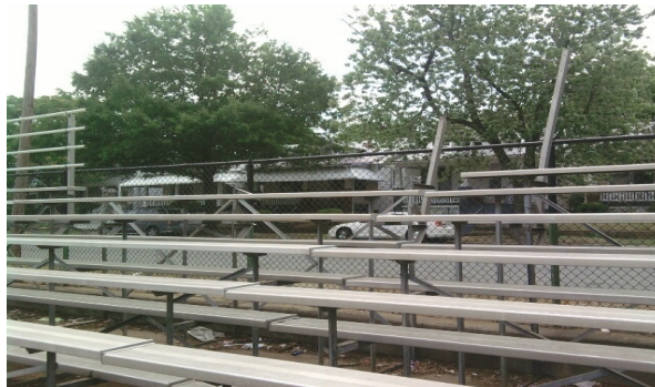
Bleachers missing back support bars at Parker Field
