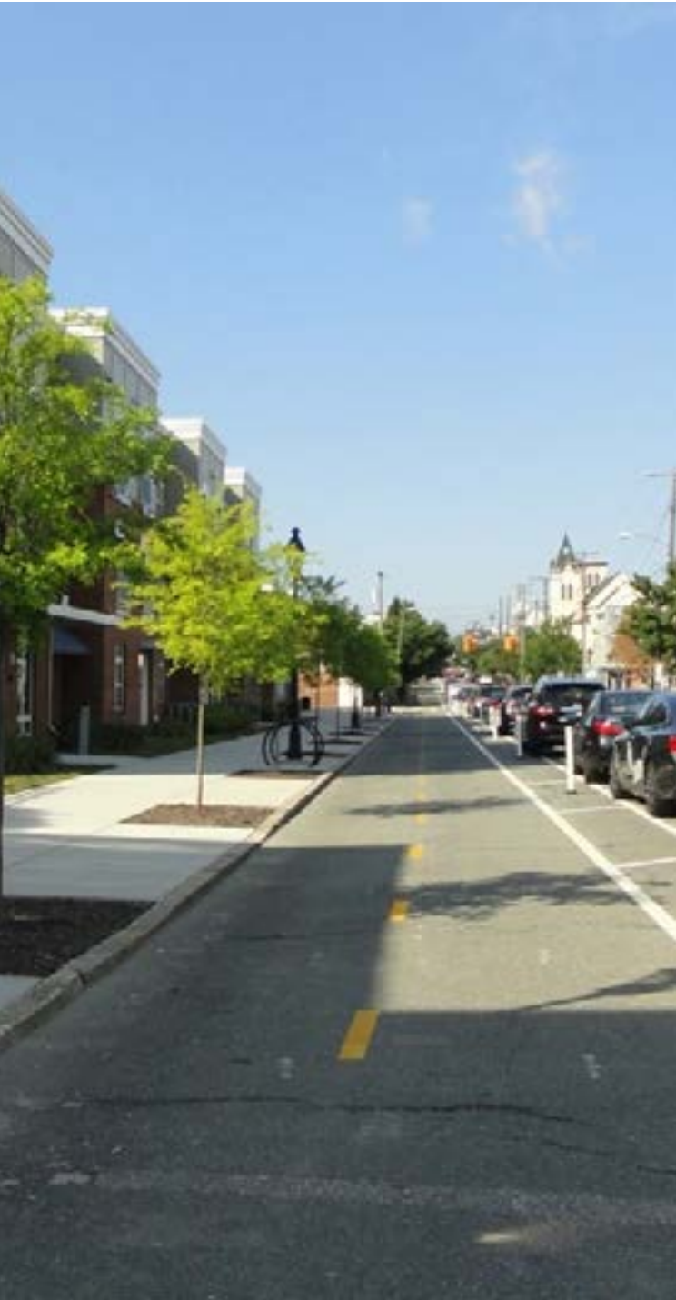
1st Street Bike Infrastructure (Credit: City of Richmond, VA)
