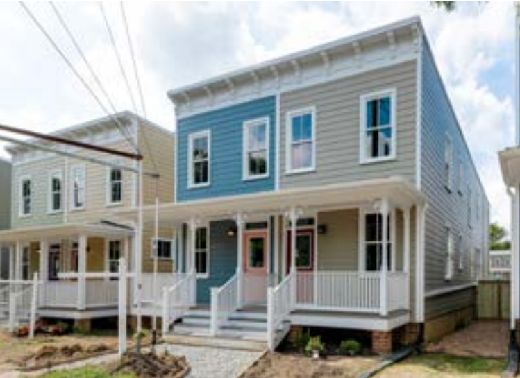
Duplex on Solar Row (Source: Mick Anders)
