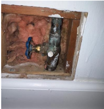
Drywall or other material covers entry point.
