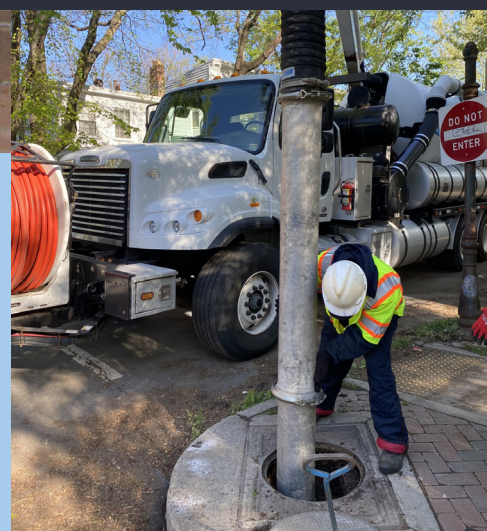
DPU employee cleaning a storm drain with vector truck hose.
