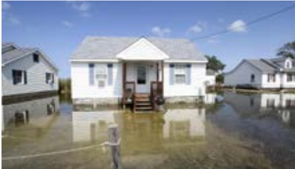
Flooded neighborhood, Richmond Department of Public Utilities
