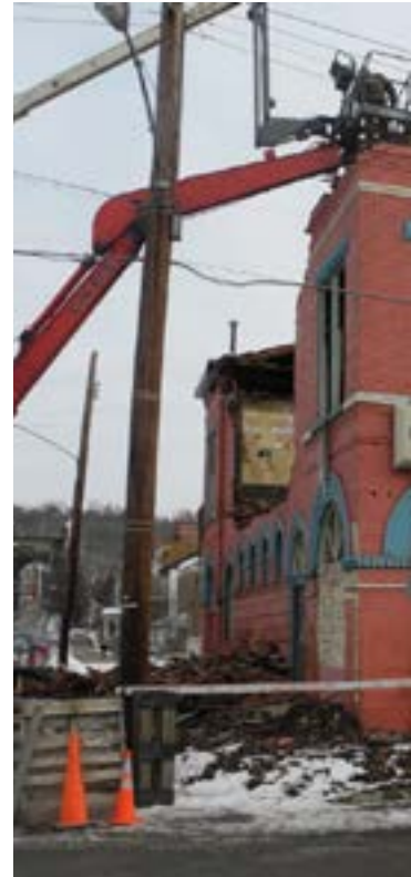
Building Demolition. CPG
