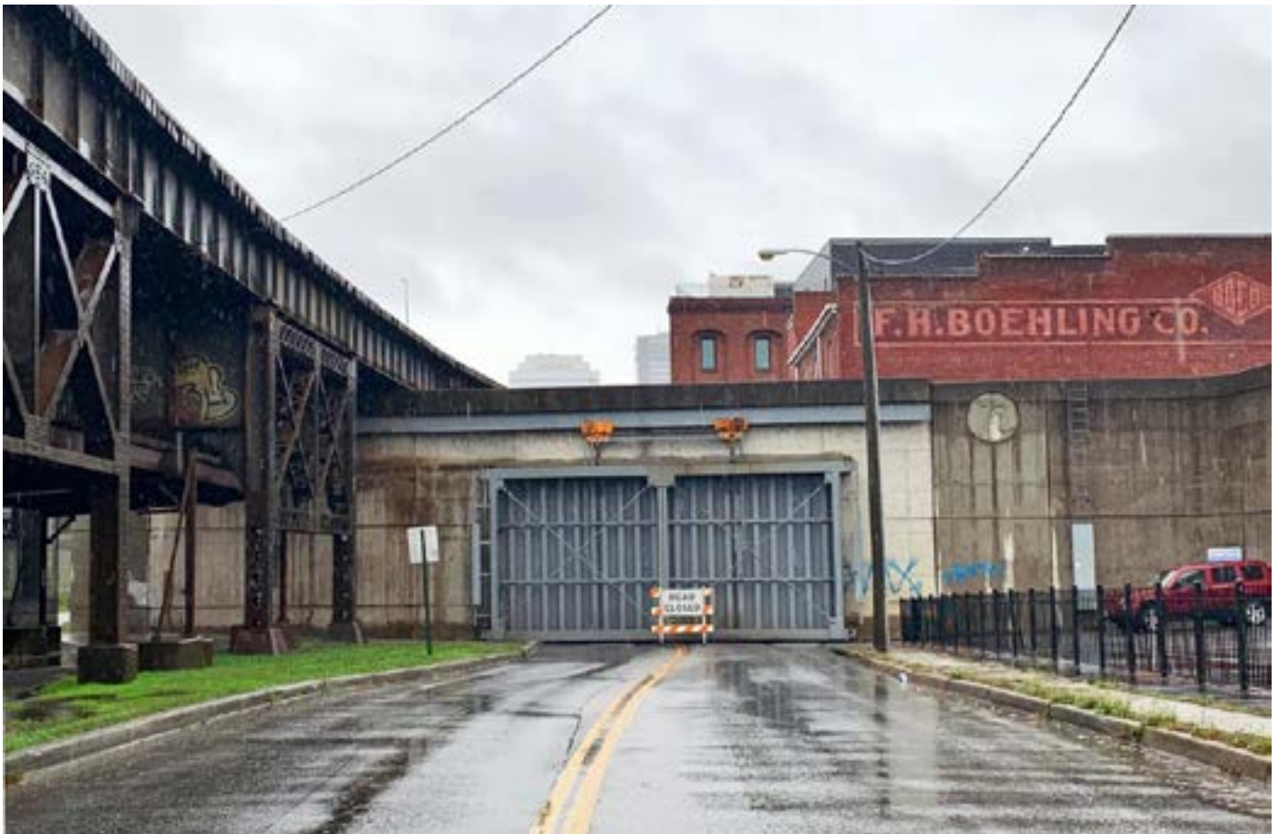
Richmond floodwall closing, WRIC
