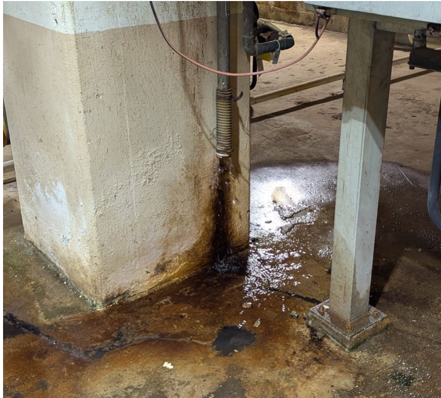
Discharging Water – Unknown Source – Plant #1 Pumping Room
