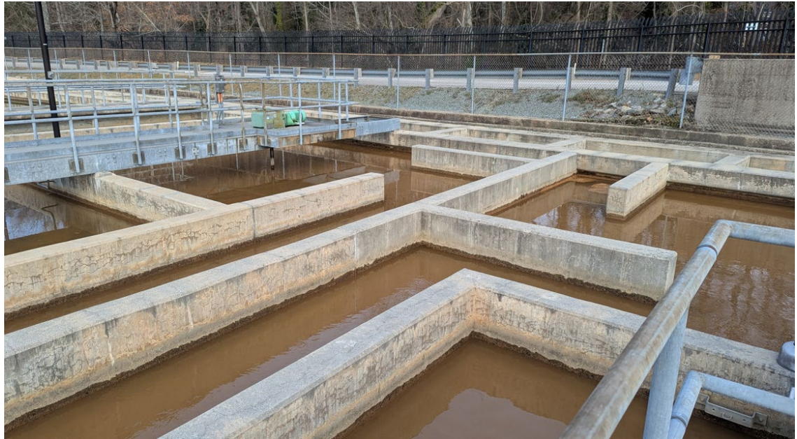
Flocculation Basins – Plant #1
