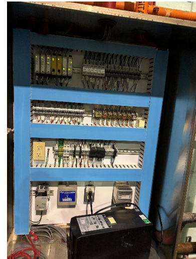
Pump Control Panel Interiors
