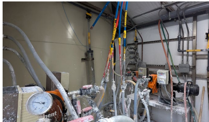
Lime Slurry Tank and Feed Equipment
