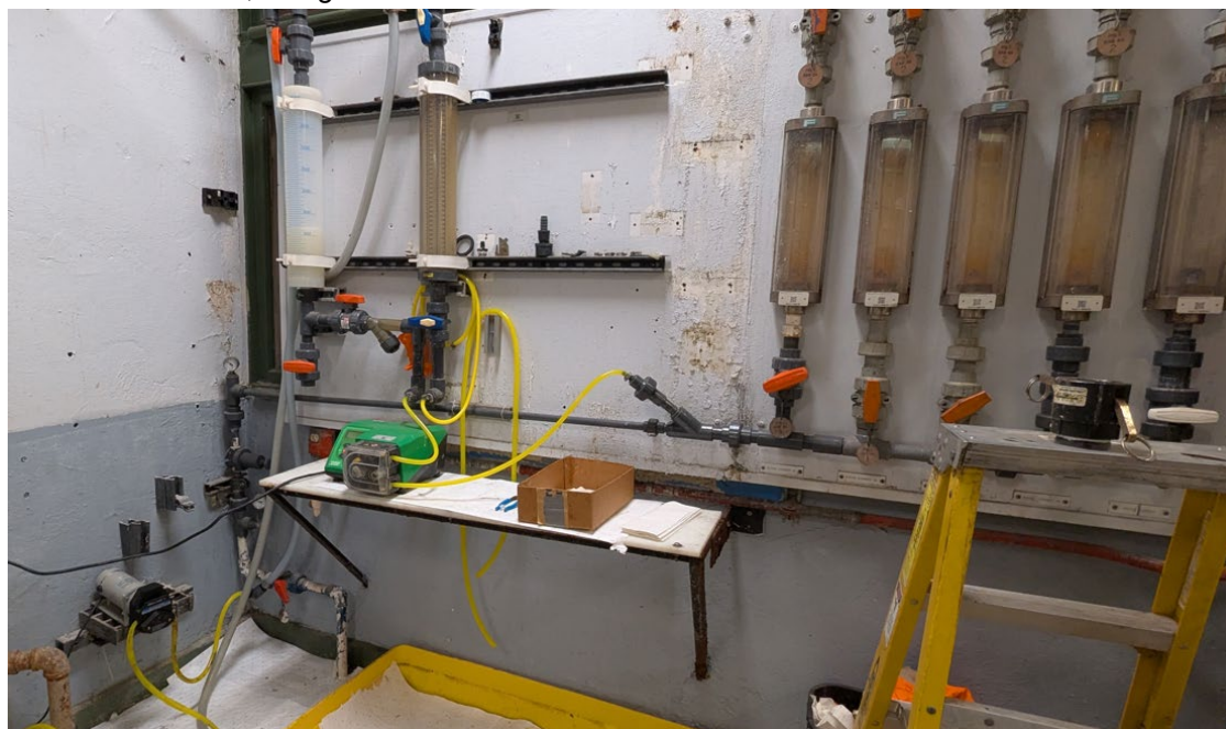
Plant #1 – Polymer Chemical Storage and Feed
