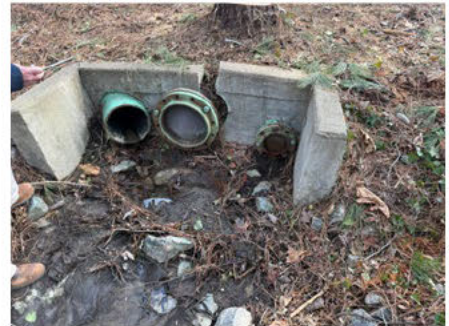
Damaged Drainage Structure
