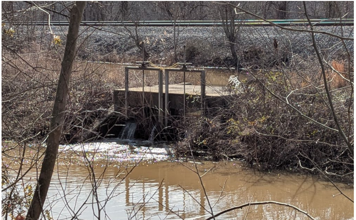
Recycled Water Inlet to Pre-sedimentation Basin
