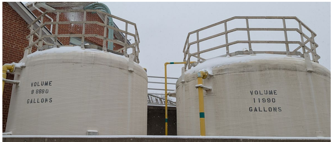
Caustic Storage Tanks – Left Tank Mislabeled
