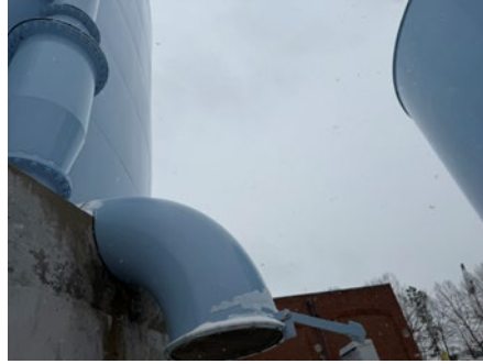
Screen Flapper Valves
