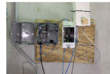
Equipment in top right of image is mounted on conduit using ziptie.
