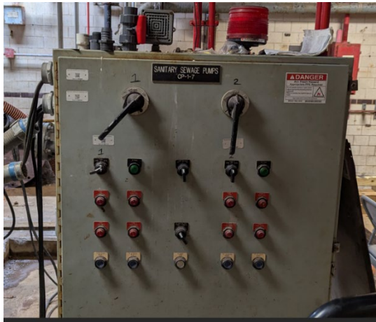
Sanitary Sewage Control Panel
