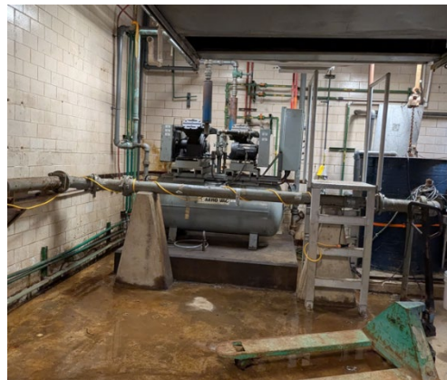
Plant #2 – Vacuum Priming System
