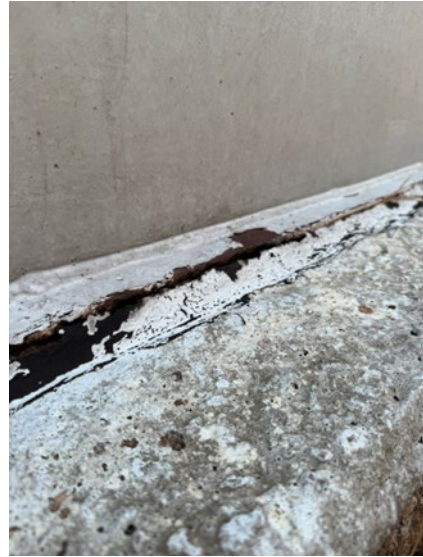
Corroded Base Plate
