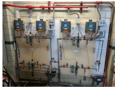
Plant #2 – Applied Water Chlorine Analyzers
