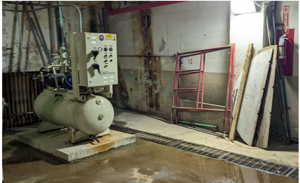
Plant #1 – Vacuum Priming System
