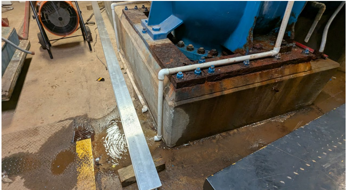
Discharging Water – Filtered Water Pump S4 (Plant #2)
