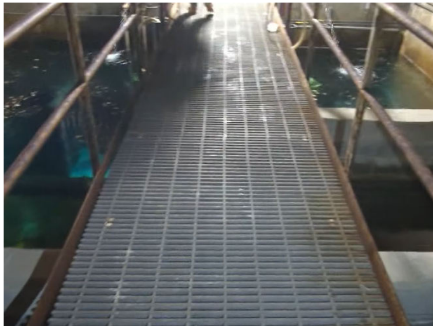
Catwalks in Chlorine Contact Basin
