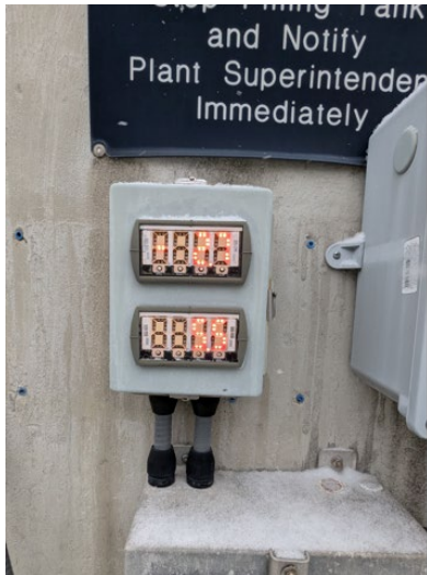
Caustic Storage Tank Level Indicator
