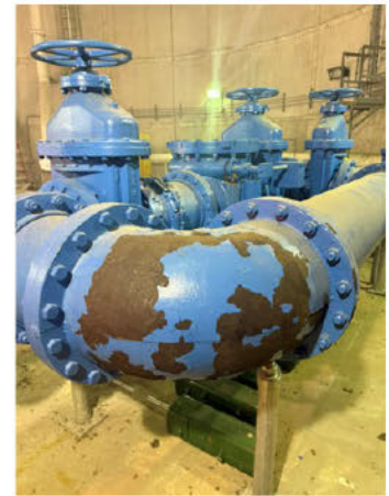
Damaged Process Piping Coating
