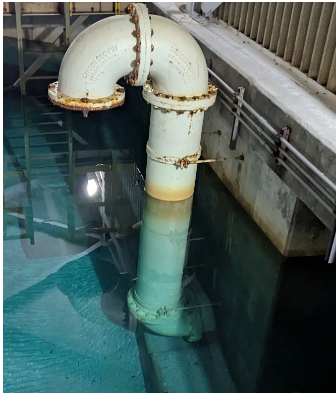
Filter Plant #1 Vent into Chlorine Contact Basin
