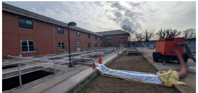
Godwin Pump Suction Piping
