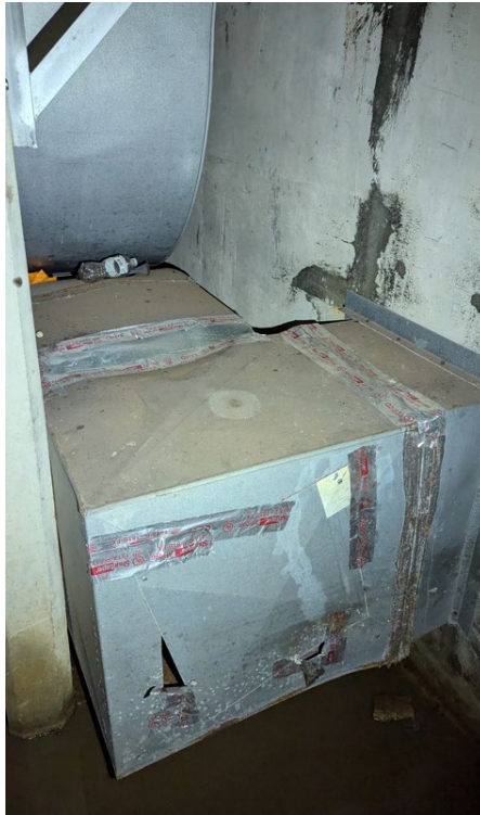
Wastewater Pumping Station Damaged Ducts and Heating Control Panel
