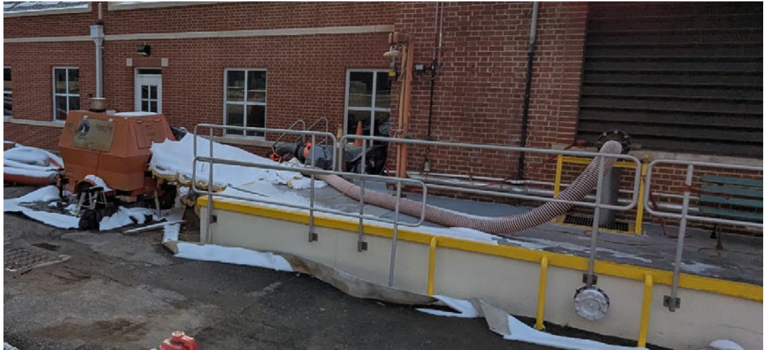
"Godwin" Portable Dewatering Pump – Plant #1
