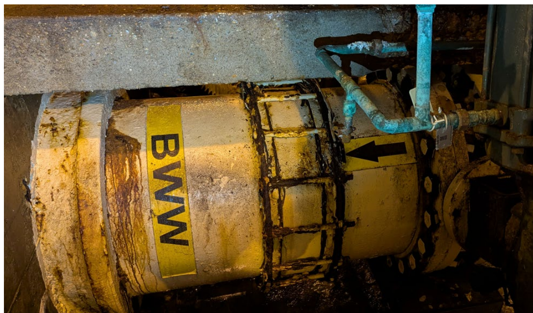
Backwash Waste Water Piping in Plant #2
