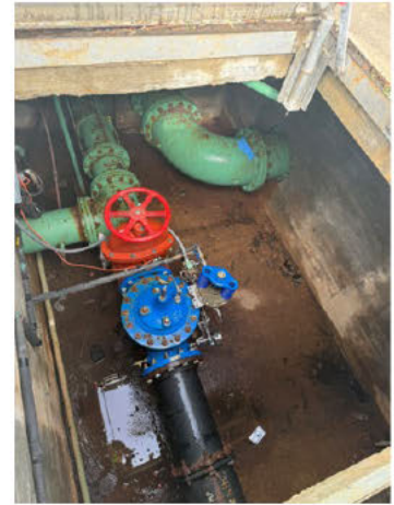
Altitude Valve Vault
