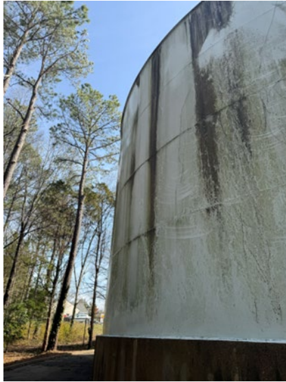
Mildew on Tank Exterior
