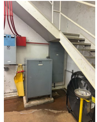
Water Pooling Around Electrical Equipment
