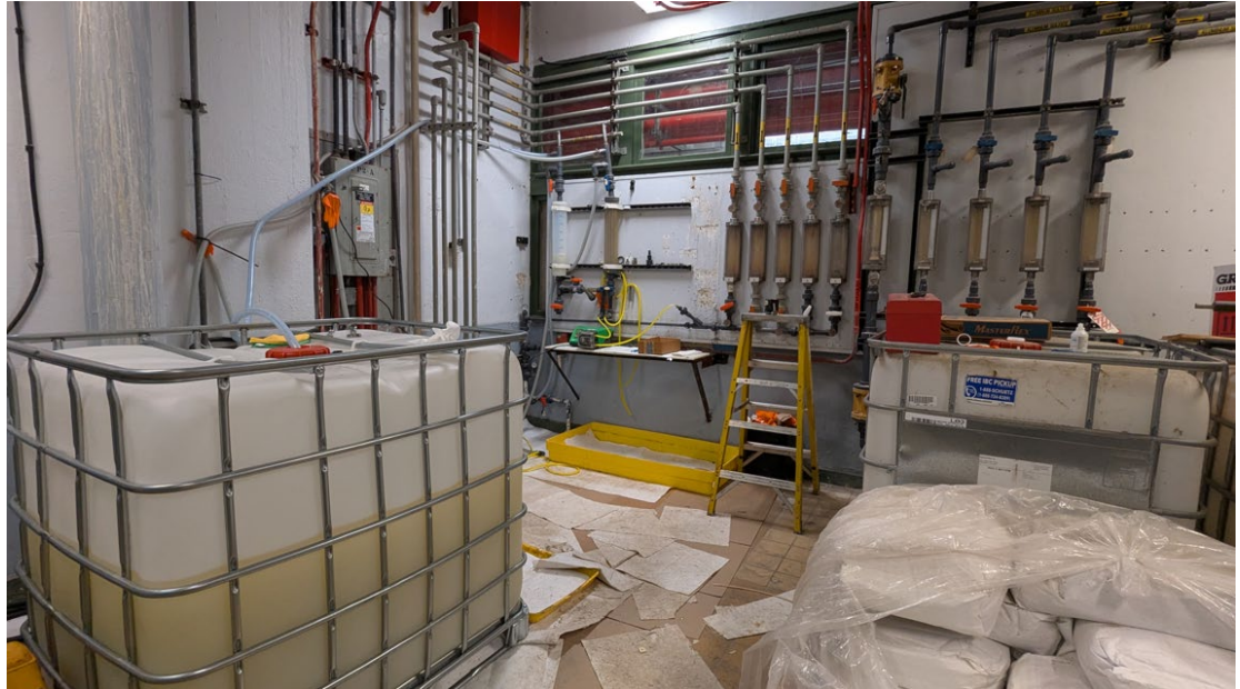
Plant #1 – Polymer Chemical Storage and Feed
