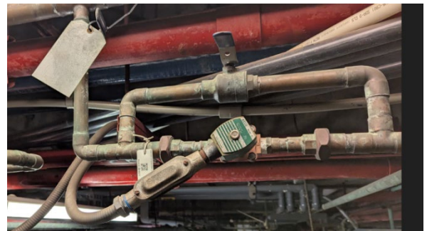
Plant #2 – Vacuum Priming Solenoid and Bypass
