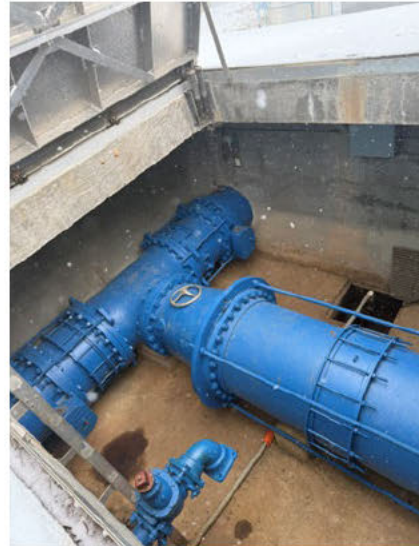
Vault Process Piping
