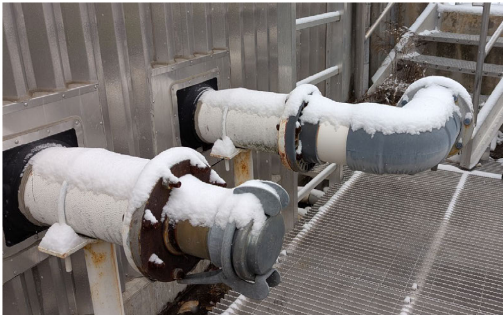
Plant #1 – Drain Suction and Discharge Connection
