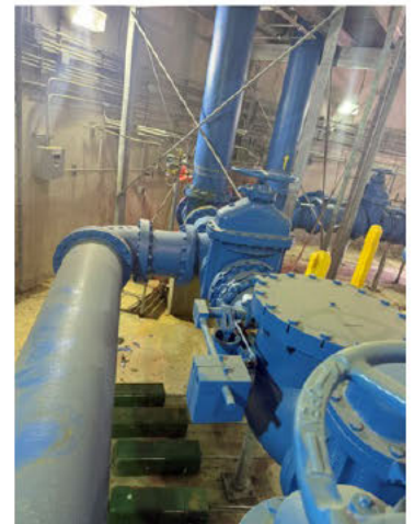
Effluent Line Swing Check Valve
