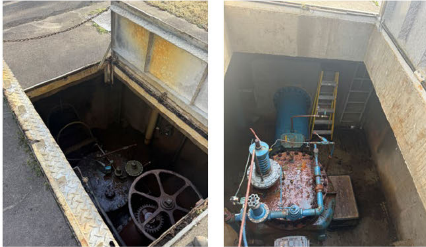
Altitude Valve Vaults
