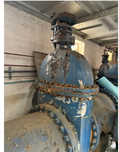
Combined Discharge Header with Excessive Corrosion
