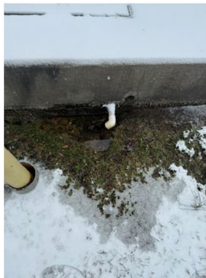
Sump Pump Discharge
