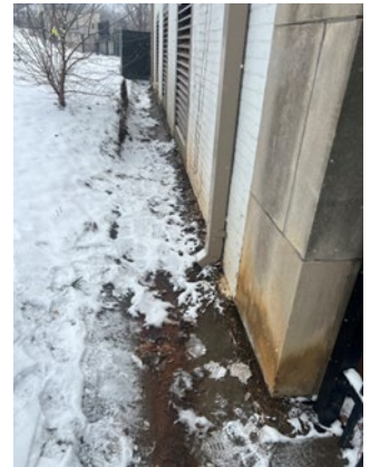
Water Staining on South Side
