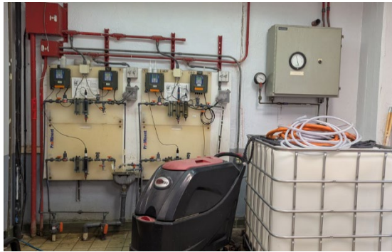
Plant #1 – Applied Water Chlorine Analyzers
