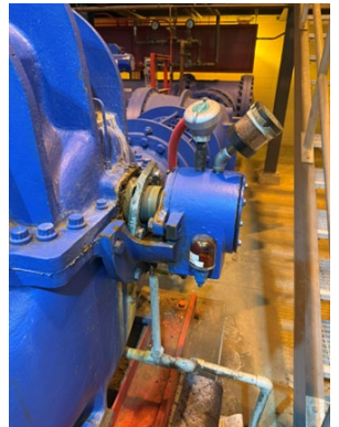
Missing Shaft Cover
