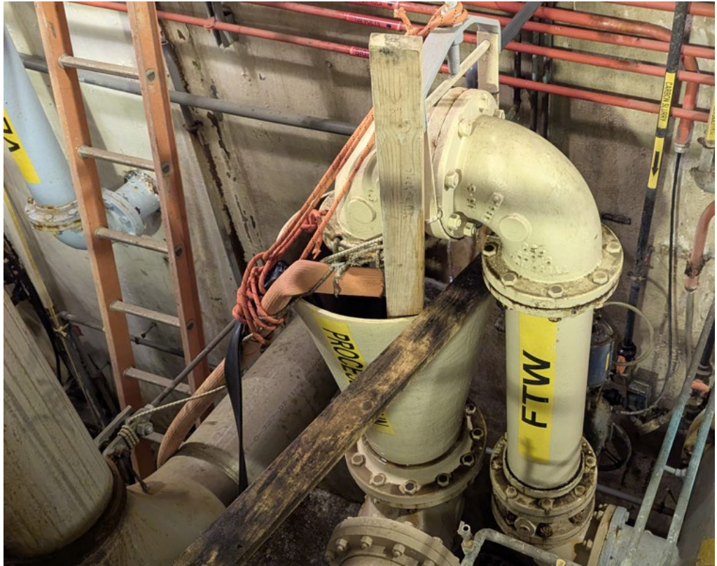
Sump Pump Hoses Routed to Additional Process Drains – Plant #2
