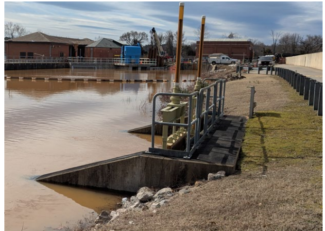
North Basin Intake Gates – From Pre-sedimentation
