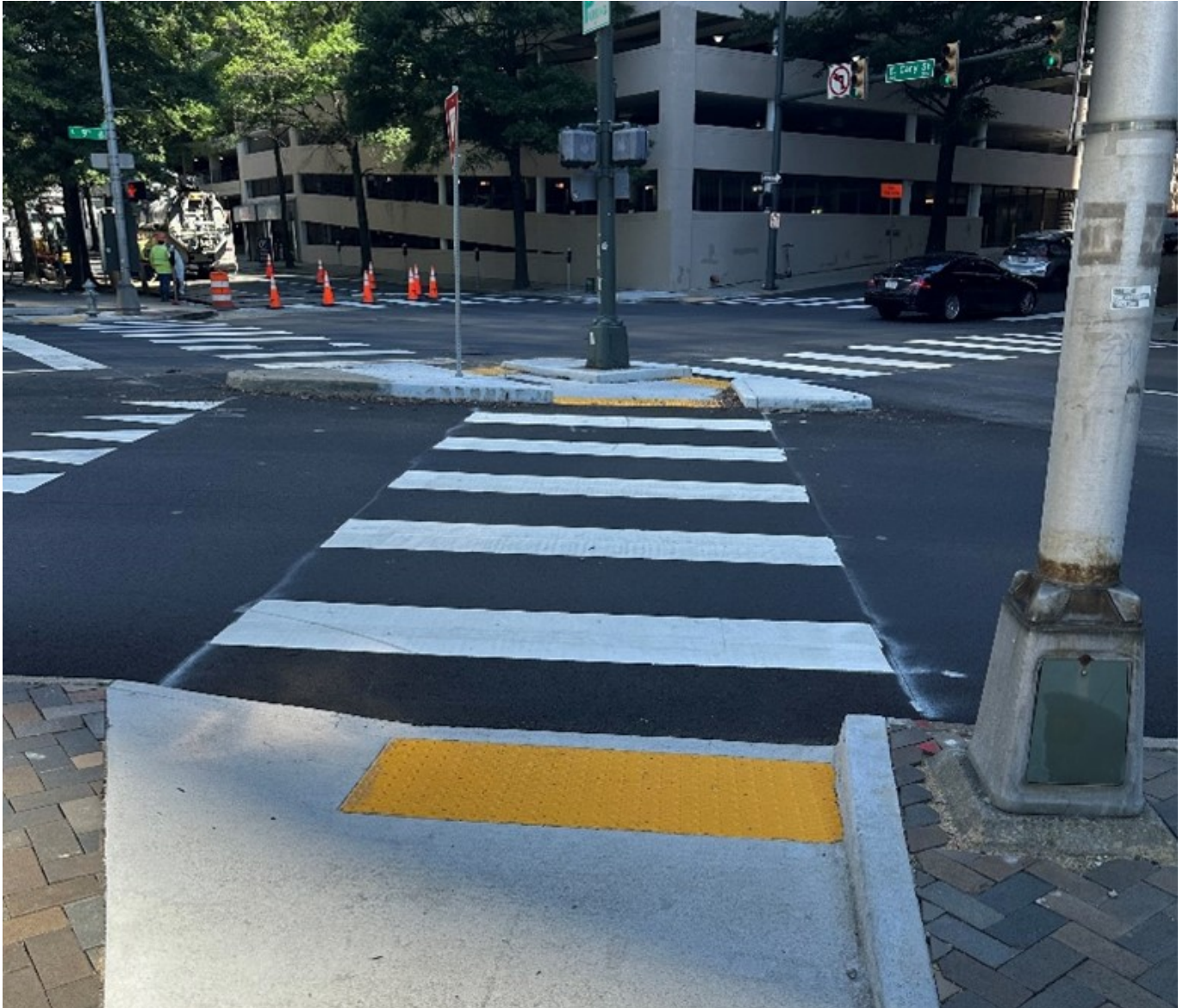
Pedestrian Crossing at the intersection of Cary Street and 9 th Street.
