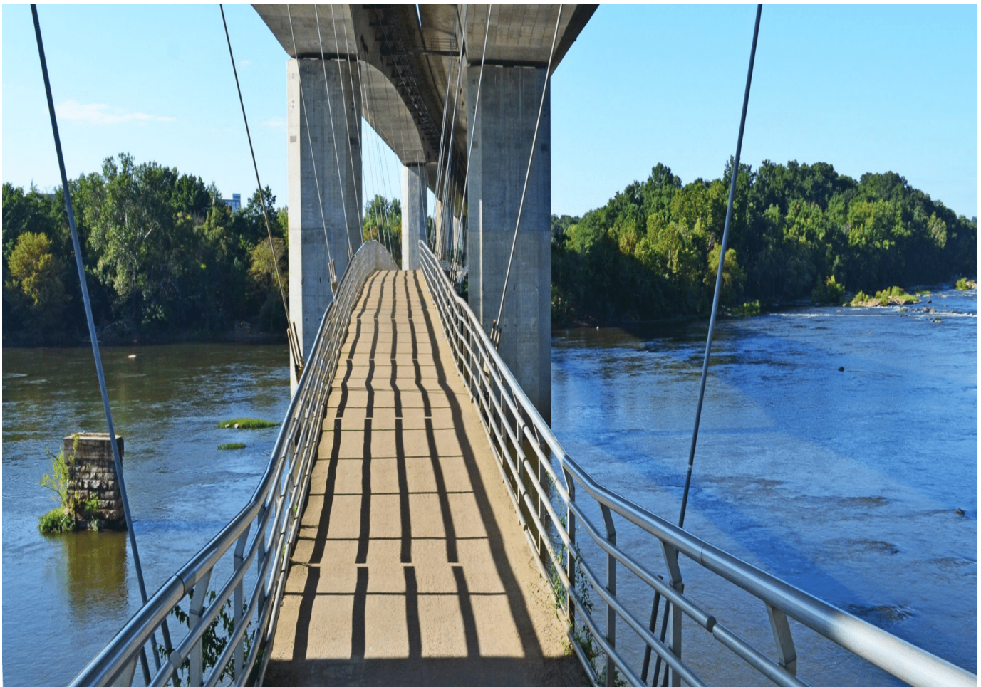
View of the James River from the Belle Isle Suspension Bridge.
