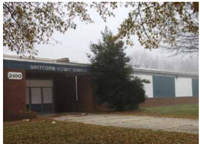
Former Whitcomb Court Elementary School demolished 2016
