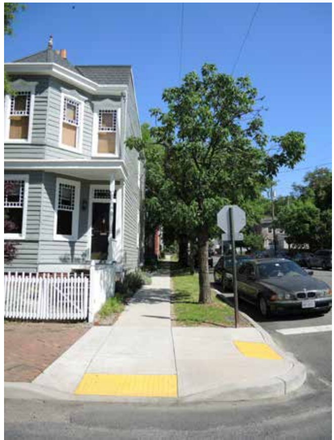
A new sidewalk in Church Hill includes ADA-compliant ramps at the intersection.
