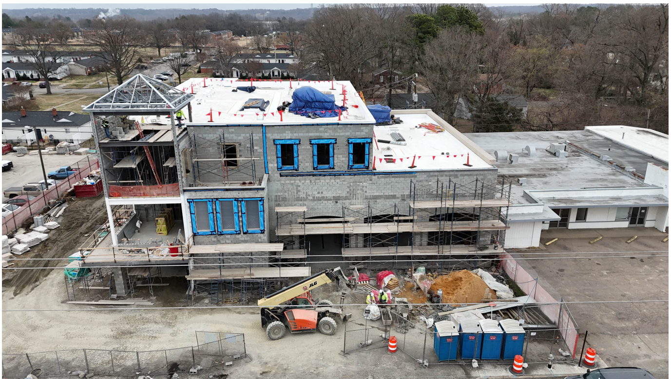
Ongoing construction, Fire Station 21.
