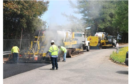
Heat Scarification Operation
