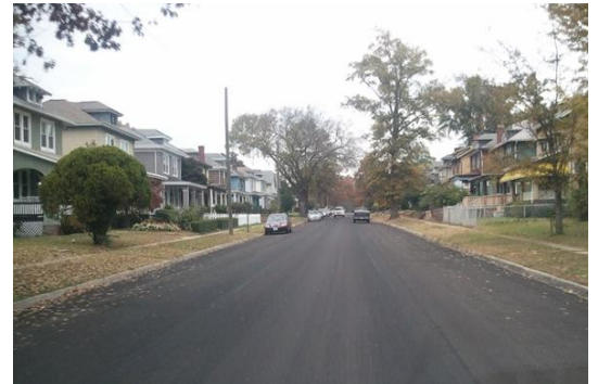
Completed Slurry Seal Application
