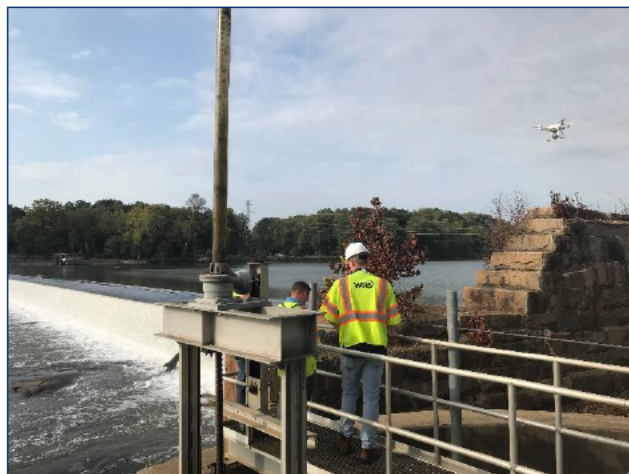
Photo 2: Drone Inspection of Boshers Dam
