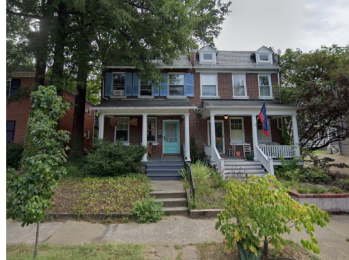
409 / 411 Tilden St - Stairs & Porch
