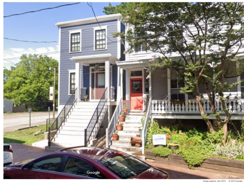
720 Jessamine St - Stairs & Porch
