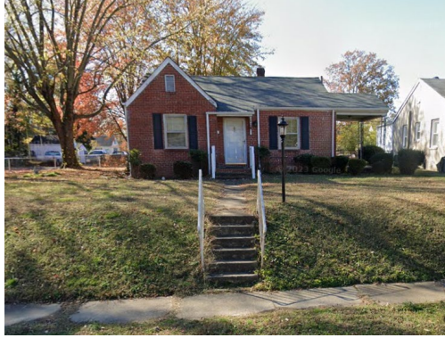
106 E 35th St - Stairs and Stoop
