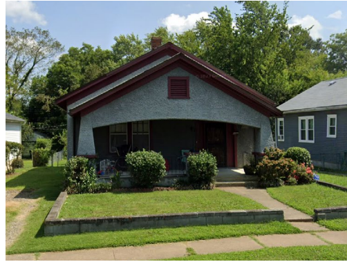
2106 Fairfax Ave - Porch
