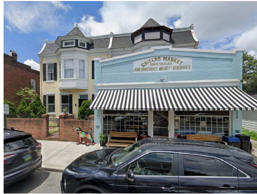
206 N Shields Ave - Shopfront
