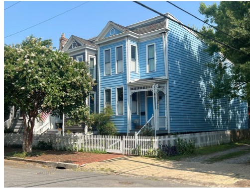
2212 M St - Stairs & Porch
