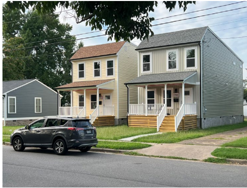
708 & 710 Cheatwood Ave - Stairs & Porch
