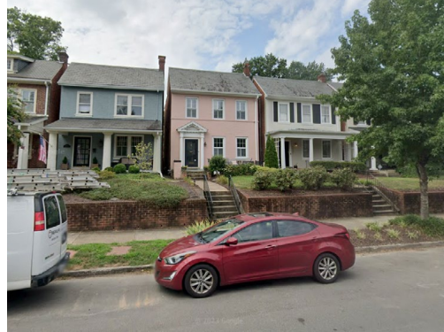
3225 Kensington Ave - Stairs & Stoop
