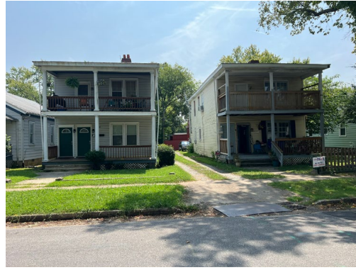
2114 & 2116 Fairfax Ave - Porch & balcony
