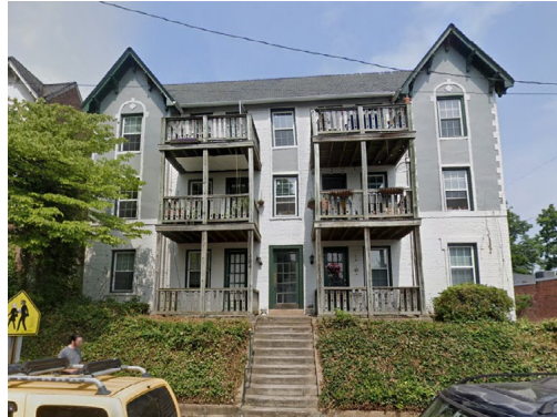
404 Cleveland St - Stairs, Porch, & Balcony
