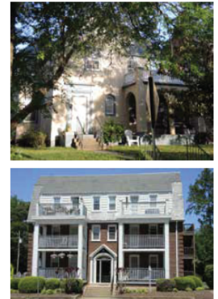
Duplexes, also known as two-family homes [top], and small multi-family buildings [bottom] are secondary uses.
