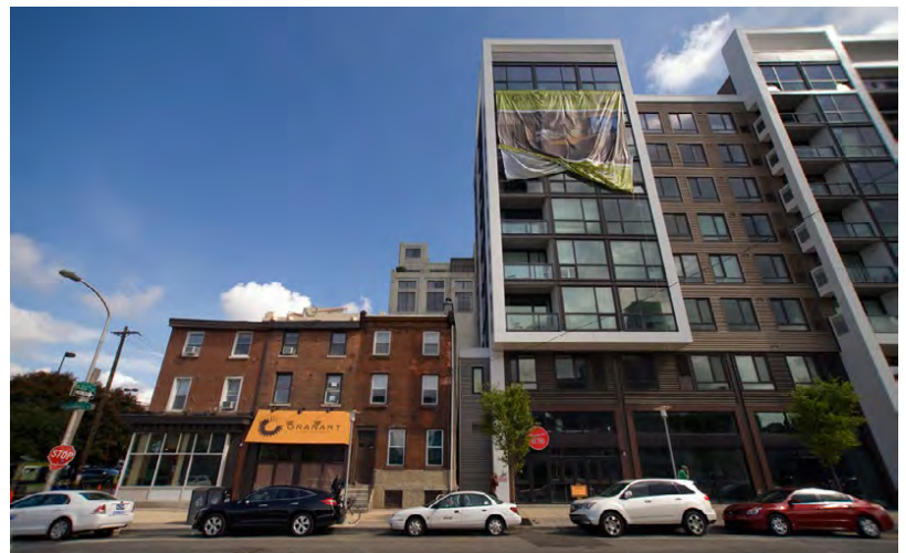
Large-scale infill, Philadelphia, PA, Bradley Maule
