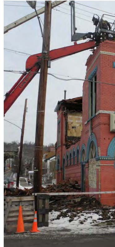
Building Demolition. CPG
