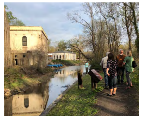
Pump House Park tour, Ellen Chapman
