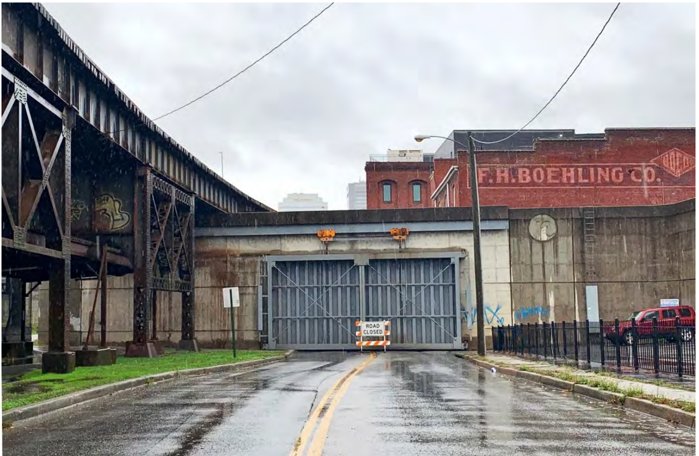
Richmond floodwall closing, WRIC
