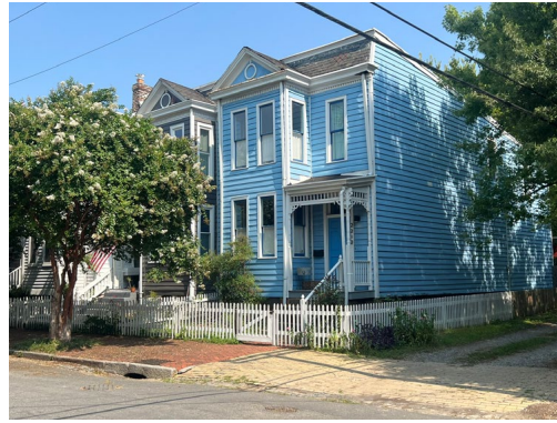
2212 M St - Stairs & Porch
