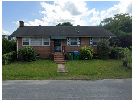
3009 V St - Stairs & Porch
