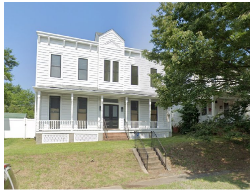
2810 Griffin Ave - Stairs + Porch
