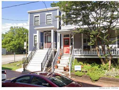
720 Jessamine St - Stairs & Porch
