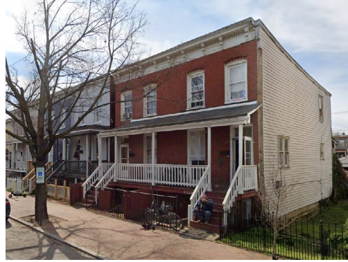
332/334 S Laurel St - Semibasement + Porch
