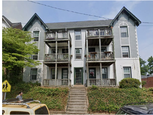
404 Cleveland St - Stairs, Porch, & Balcony
