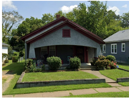
2106 Fairfax Ave - Porch
