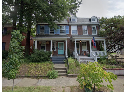
409 / 411 Tilden St - Stairs & Porch
