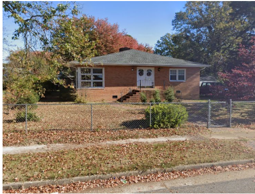
207 E 36th St - Stairs and Stoop
