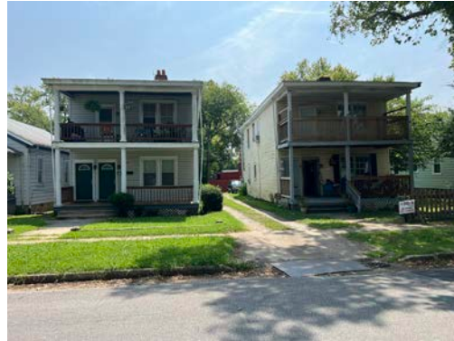
2114/2116 Fairfax Ave - Porch+balcony
