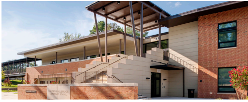
Oak Grove Bellemeade Elementary School
