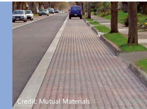
Permeable pavers in parking lane
