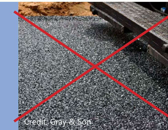
Porous asphalt is not permitted
