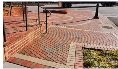
Brick is a predominate material used for Richmond sidewalks
