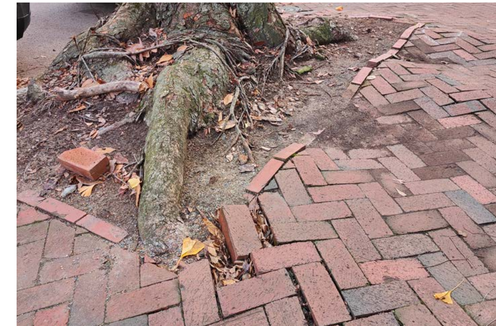
Larger, historic trees have caused the existing pavers to move due to the growth of the tree root system.
