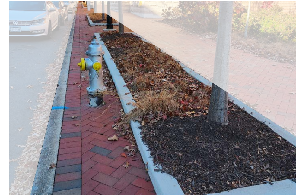
The planting bed setback from the road edge allows for a larger planting area and a ease of access for drivers exiting / entering their vehicles, but collects debris and is a tripping hazard.
