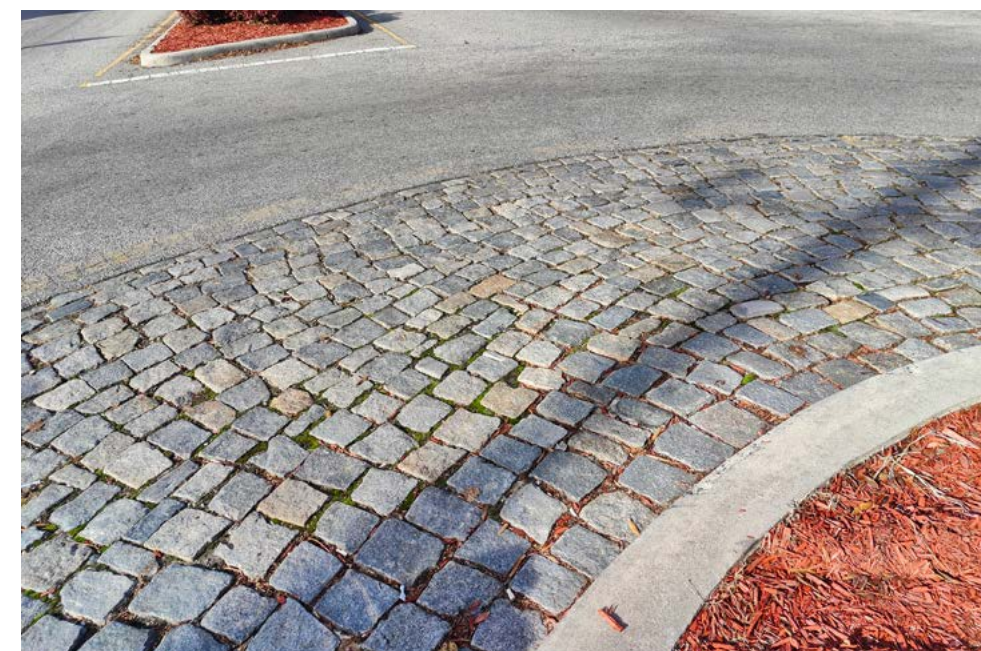
Cobblestones are periodically used as an accent material throughout Church Hill for vehicle calming and aesthetics.
