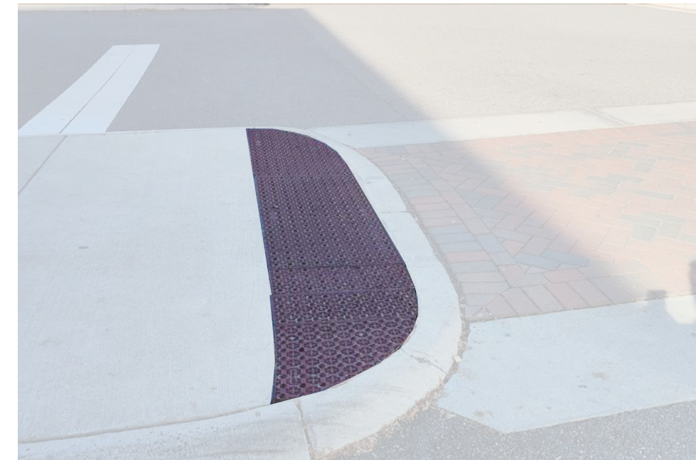
Detectable warnings visually match the surrounding character and warn users of a pedestrian crossing.
