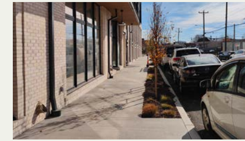
Tree wells are often long enough to hold more than one tree
