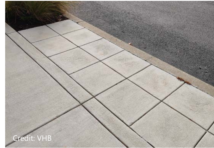
Credit: VHB Scoring pattern differentiates the Buffer and Pedestrian Travel Zones
