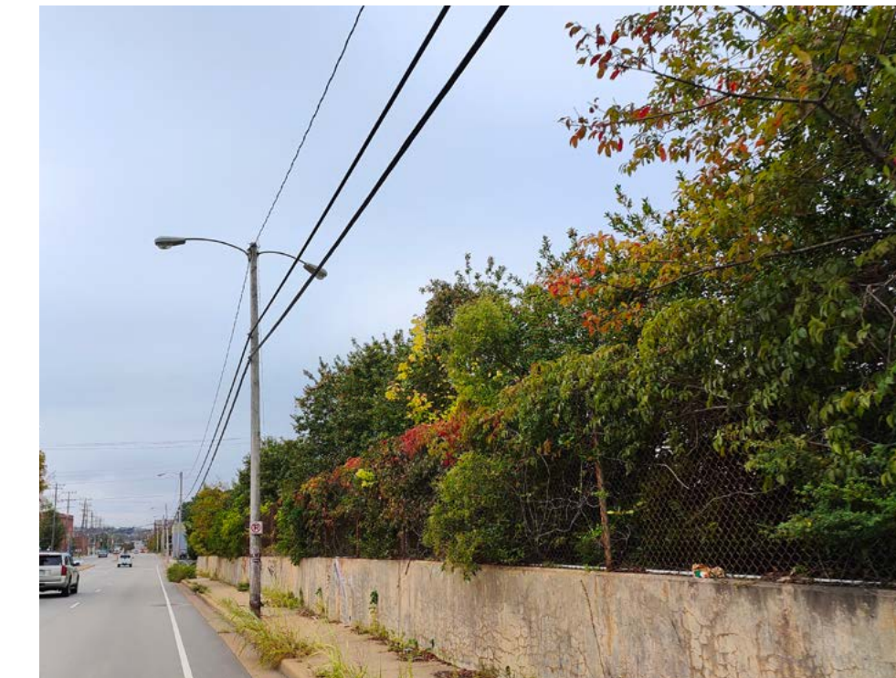
Power lines running along the existing street limit the growth potential of street trees.
