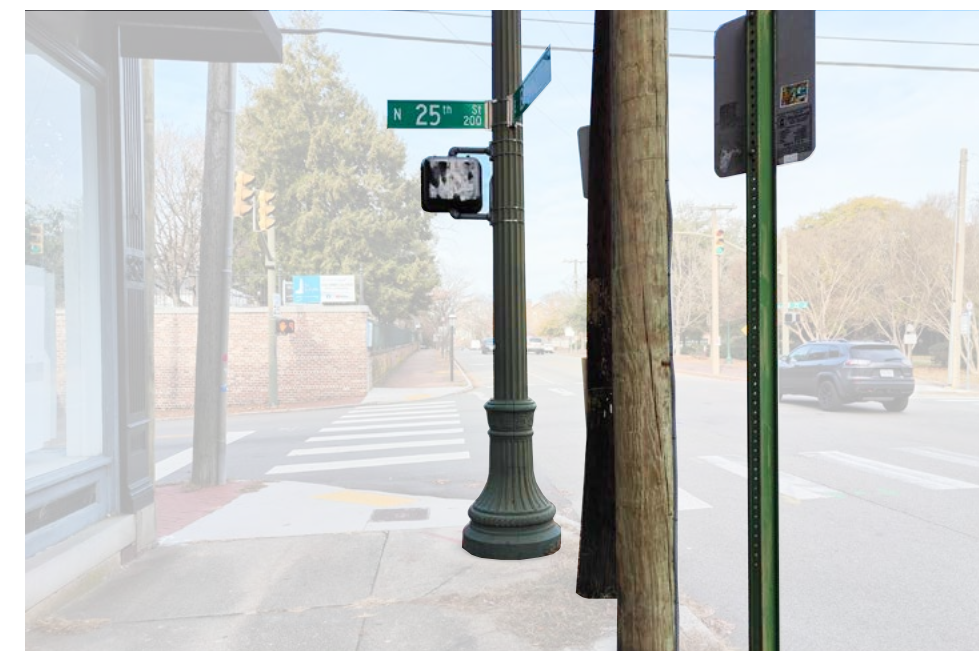
Multiple poles are evident, creating a cluttered streetscape.
