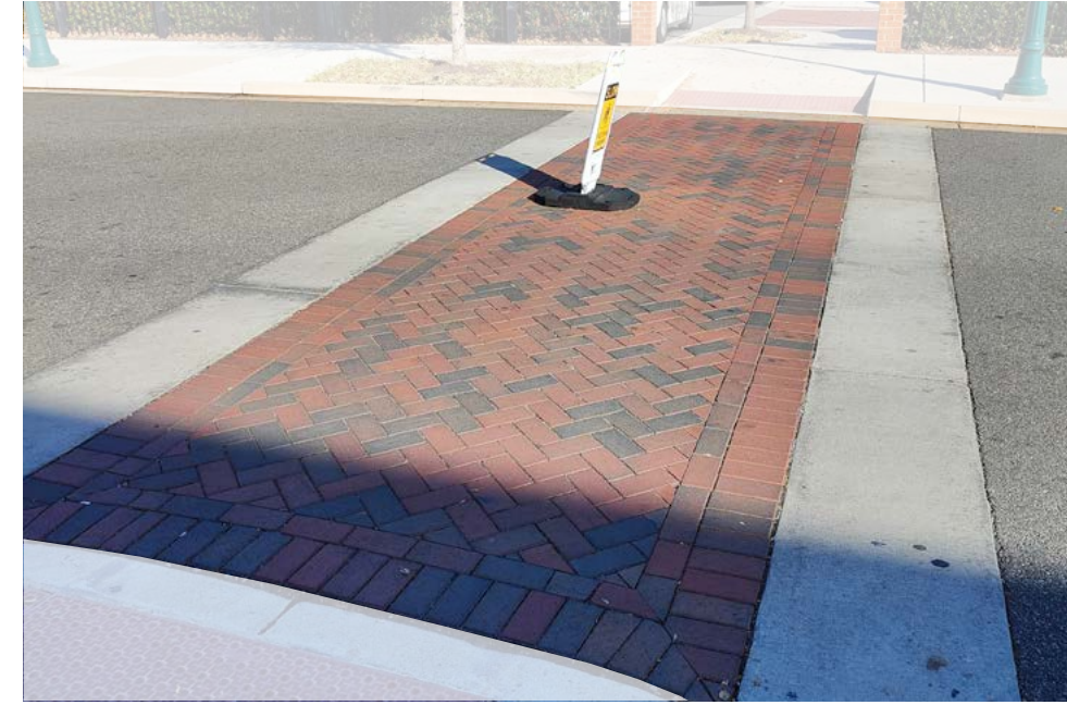
Pedestrian crossings are constructed with brick pavers and concrete borders to differentiate against the asphalt.
