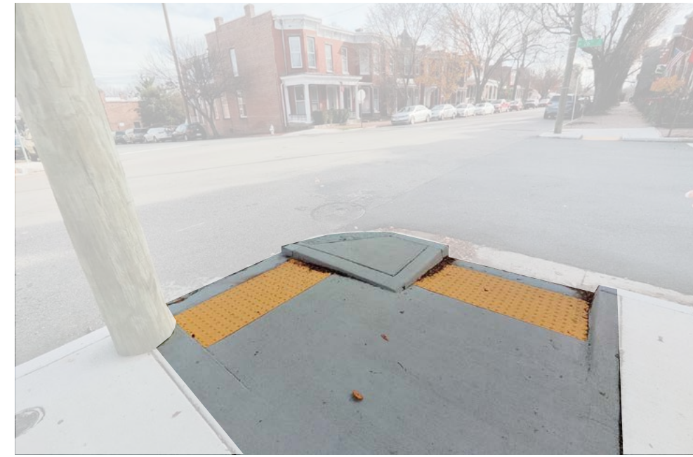
Pedestrian crossings are split to align with the parallel sidewalks. These two curb ramp crosswalks are the City of Richmond's new standard.
