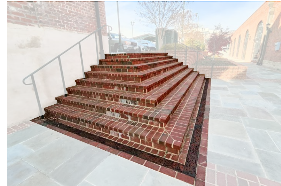
Steps and staircases are constructed with brick pavers to match and respect the surrounding built environment.
