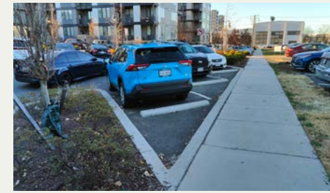
No clear distinction between sidewalk and Buffer Zone.
