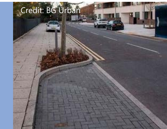
Permeable pavers in parking lane
