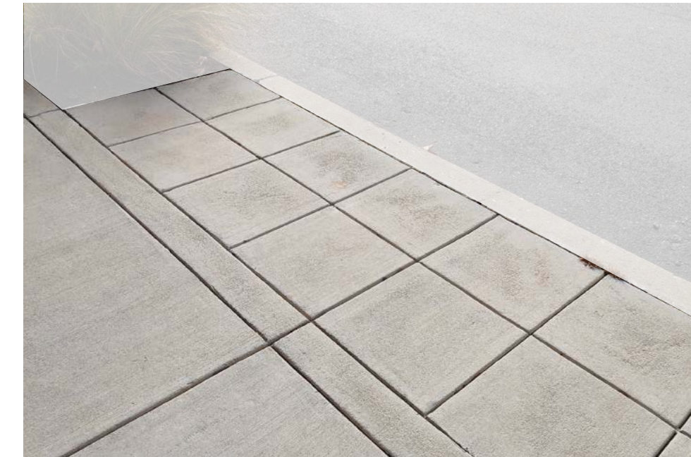
The Buffer Zone is clearly distinguished by a change in score line pattern.
