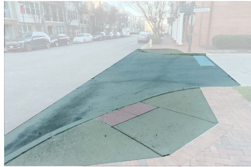
Crossings include concrete CG-12 and a concrete apron to distinguish between thoroughfare roads and side roads.
