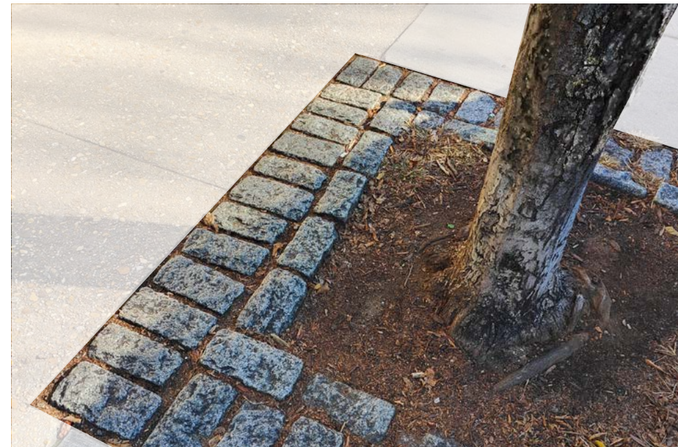
Cobblestone has been used as an accent in the planting beds for visual interest.
