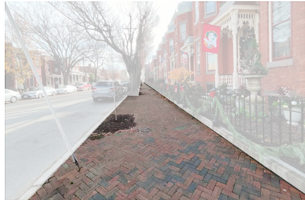
Herringbone brick sidewalks define the character of Church Hill, and are also predominant throughout the City of Richmond as a distinctive character.
