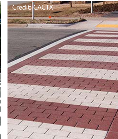
Credit: CACTX Stamped Asphalt
