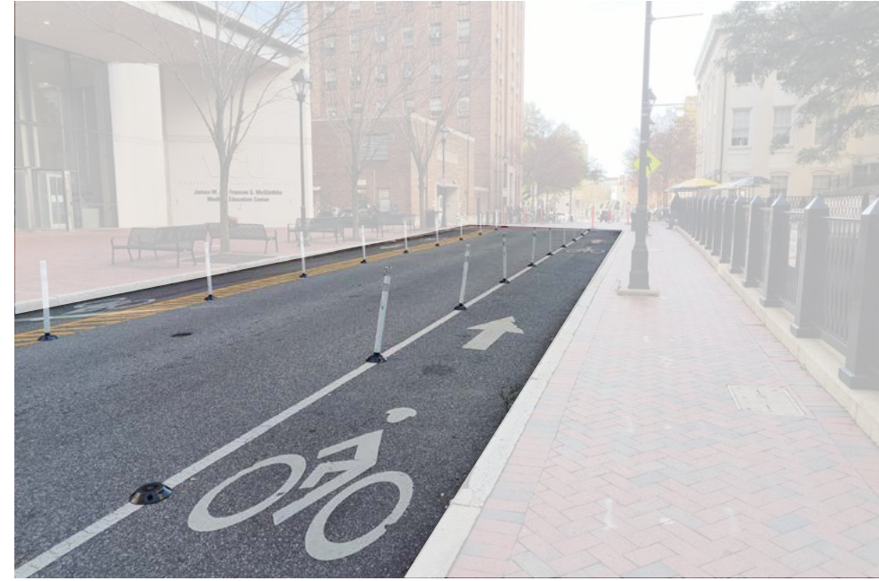
Designated bike lanes are separated from the vehicular travel lanes through traffic bollards.
