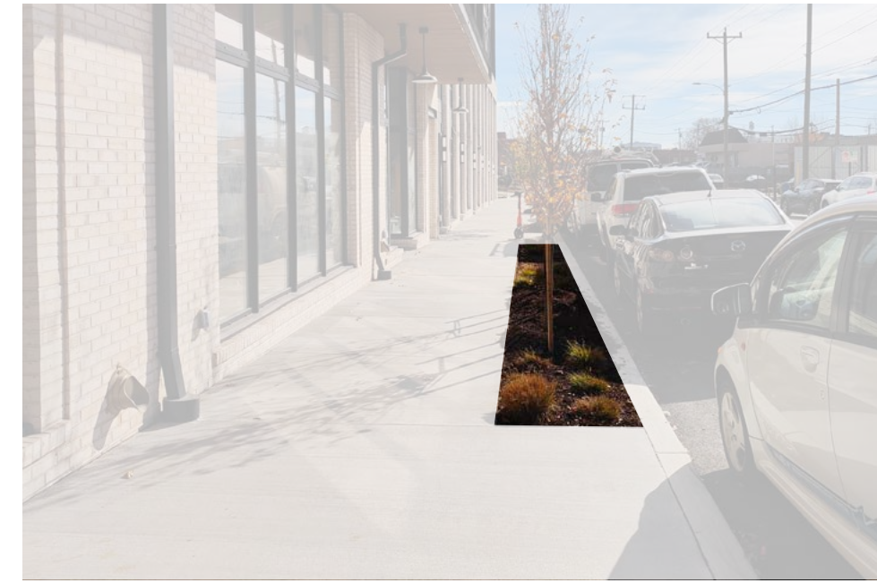
Continuous and long planting beds result in difficulty for the driver to exit their vehicle safely.
