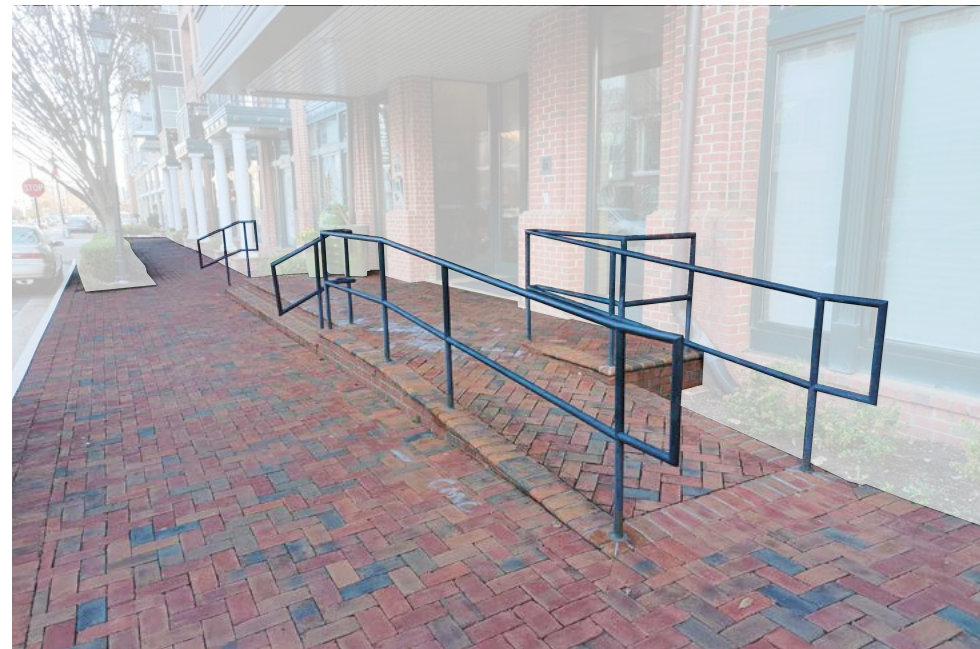
Sidewalks, stairs and ramps are all brick pavers for a consistent look, with black handrails to match architectural elements.
