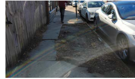
Tree wells have overgrown sidewalks
