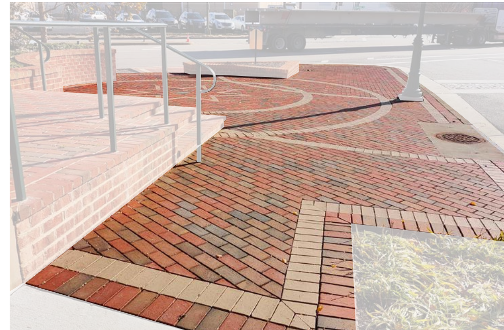
Different materials and patterns are used to provide a unique design at intersections, plazas and points of interest.
