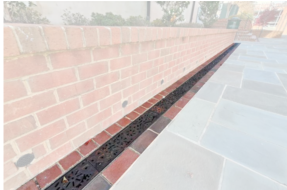
Decorative trench drains are designed to match the theme and design of the surrounding project.
