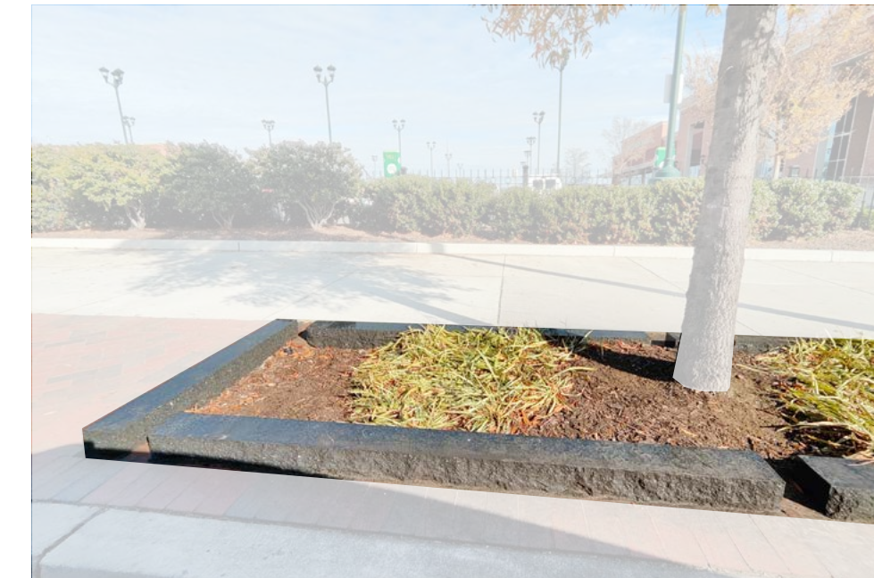
Granite curbs used for street tree wells offer visual interest, and a raised physical border to the planting beds.
