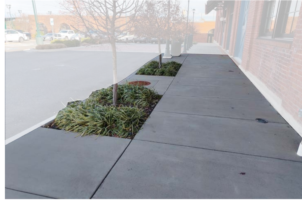
Street tree wells correspond with the score lines of the concrete. Trees and low groundcover are both planted within the wells.
