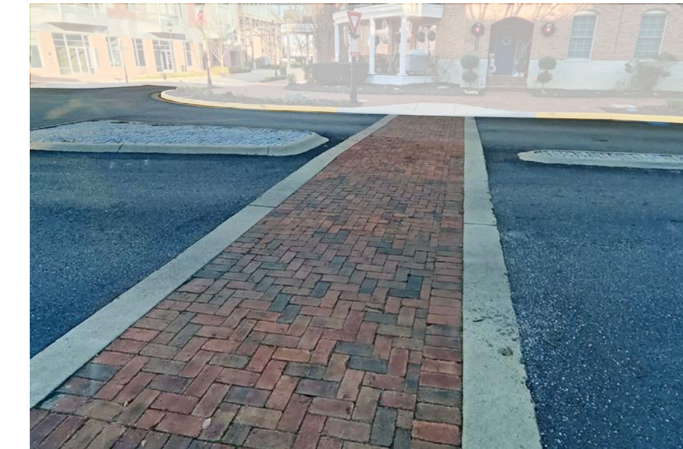
Crosswalks are brick pavers in a herringbone pattern with a concrete edge to distinguish against the asphalt drive.
