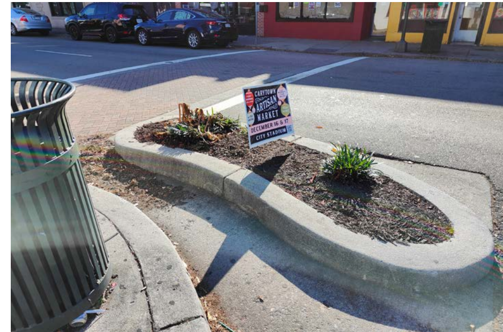
Raised traffic islands with a gutter allows for water movement but design could be adjusted to allow for large landscaping areas.
