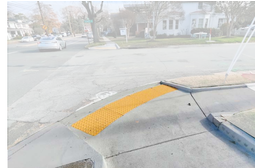
CG-12 ramp located at existing intersections.
