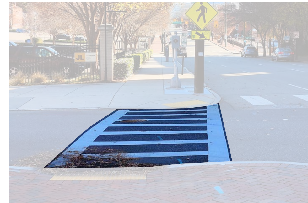
Pedestrian crossings are white ladder style with no change in elevation or material.
