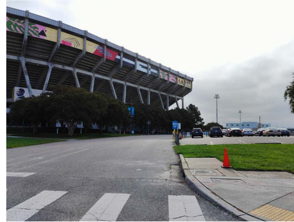
Existing pedestrian crossings include a CG-12 diagonal variation curb ramp and painted crosswalks on asphalt.
