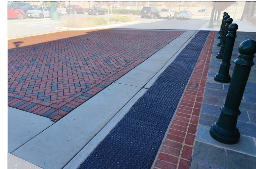
Different materials are used at junctions and pedestrian crossings to distinguish between vehicular and pedestrian zones. Detectable warnings visually match the surrounding design.
