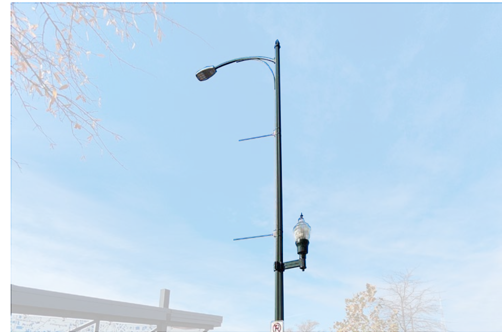
Streetlights along main thoroughfare routes have two fixture heads for both traffic and pedestrians.
