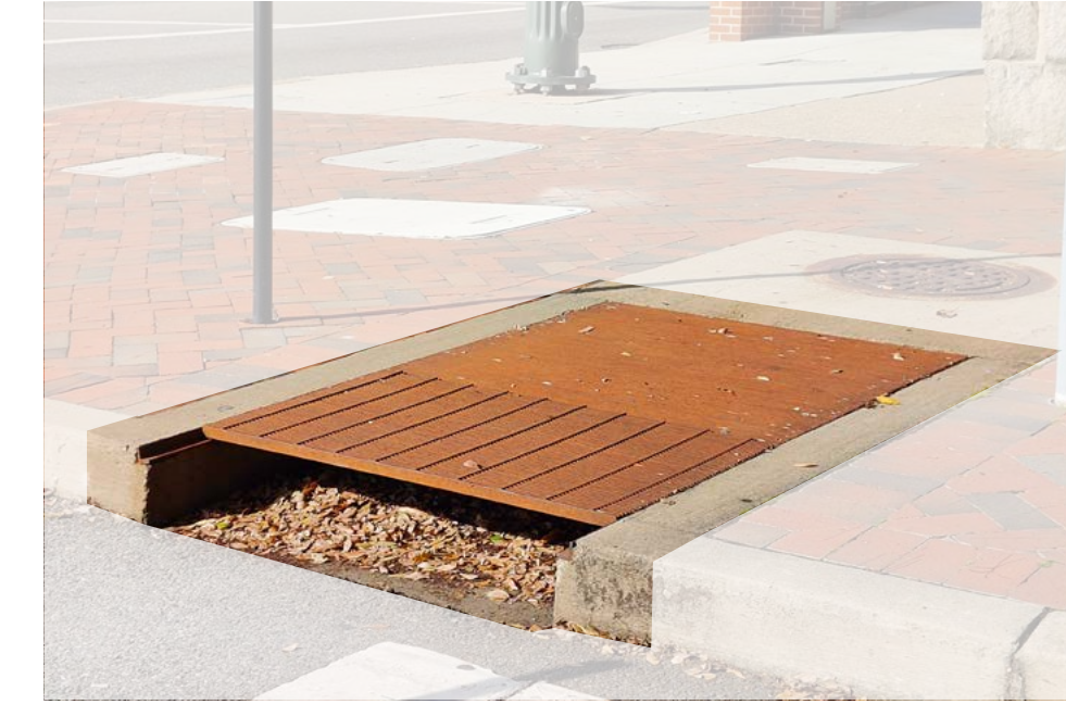
Corten steel is used for storm drains to offer a unique aesthetic to the streetscape.
