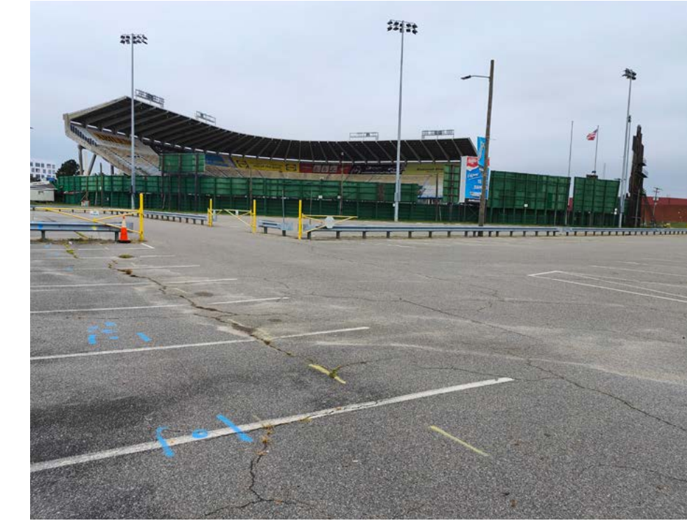
No landscaping, edge treatment, or design code has been applied to the surface parking lot.
