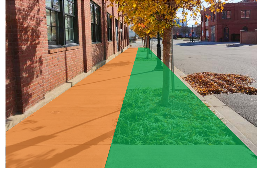
Narrower sidewalks are designed to offer a clear Pedestrian Travel Zone, a defined Buffer Zone, but no Frontage Zone.
