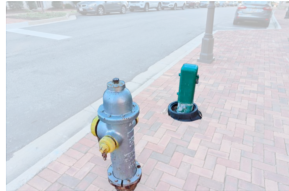
Utilities are located within the Pedestrian Travel Zone, with no screening, resulting in obstructions for users.
