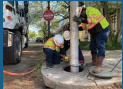
Stormwater storm drain vacuum process
