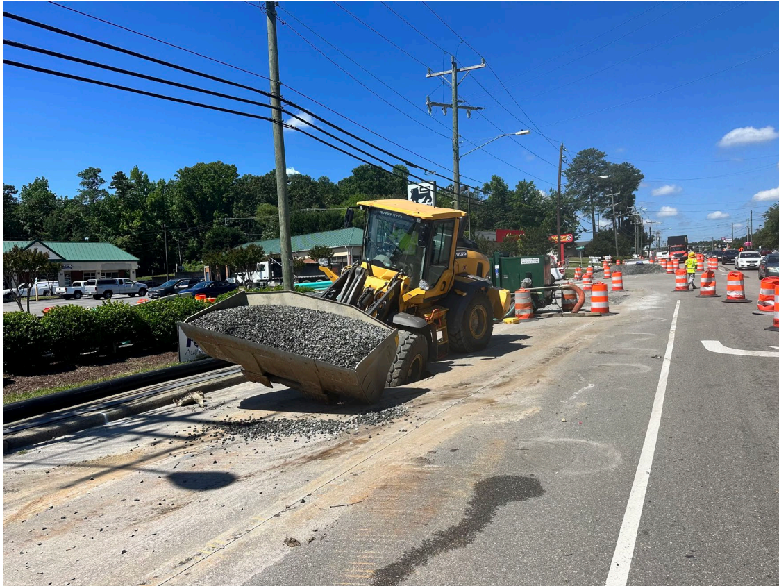
Roadway collapsed under loader with bucket of stone along LS 10 and uncovered second sinkhole
