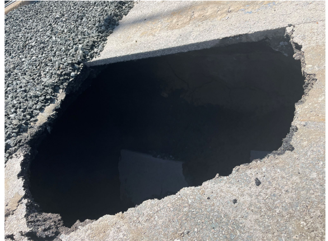
Roadway collapsed under loader with bucket of stone along LS 10 and uncovered second sinkhole
