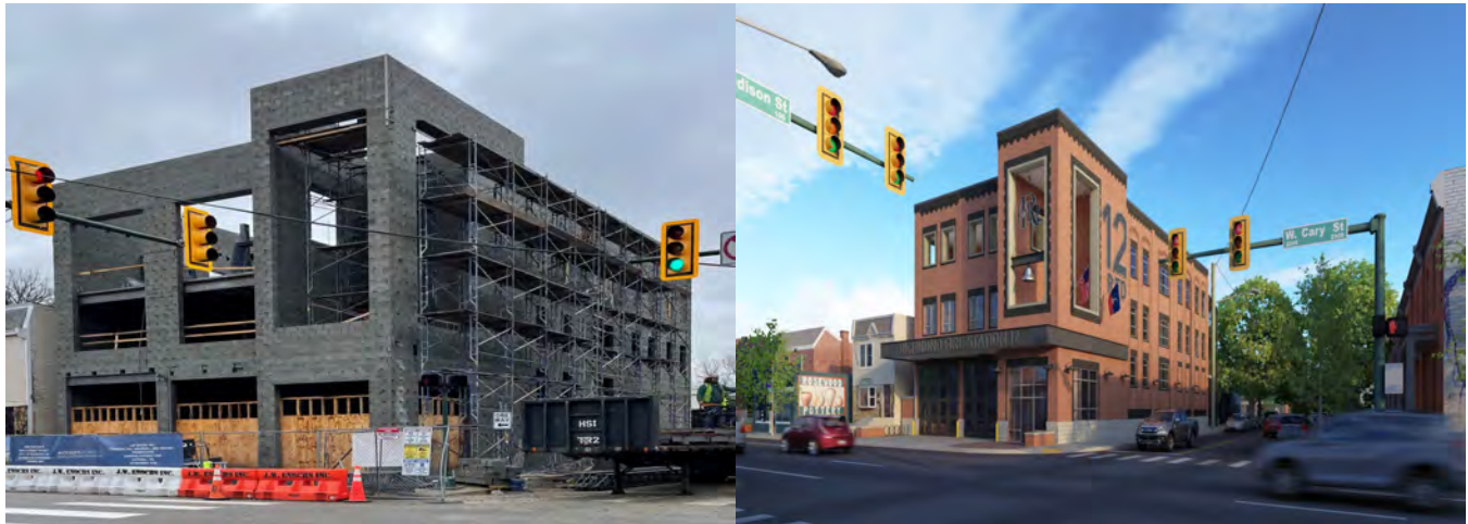
Left: Construction of Fire Station 12, as of December 29, 2023. Right: Rendering of completed building.
