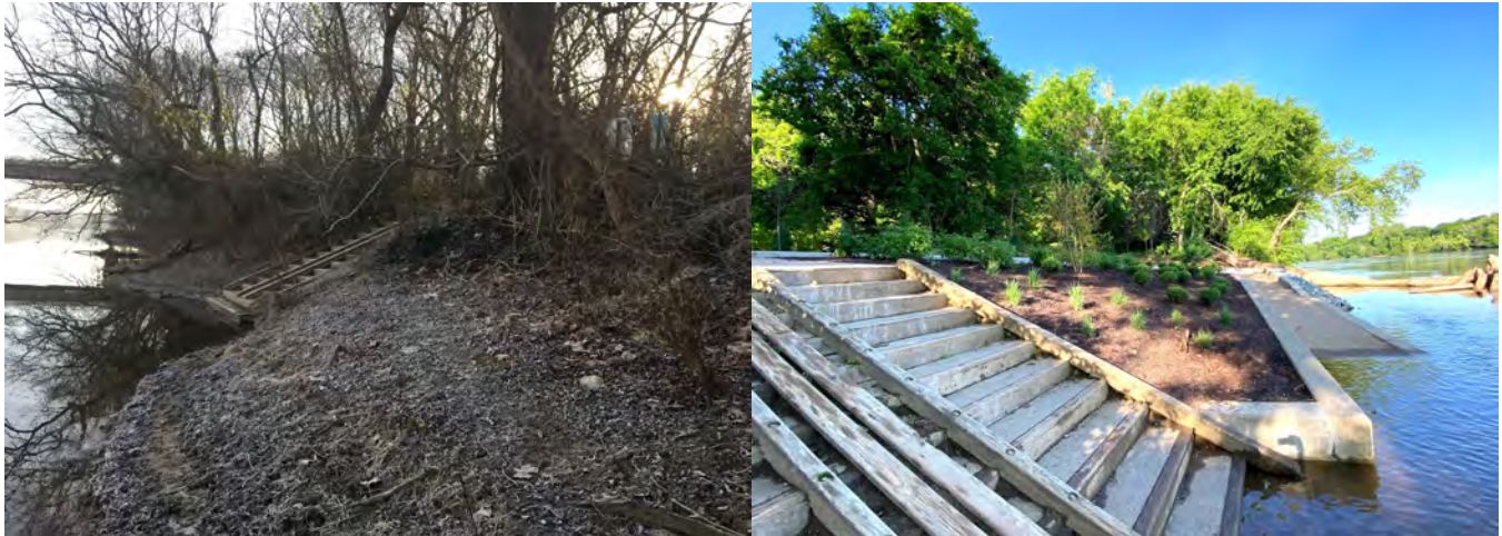
Universal Access project, before (left) and after (right) construction.
