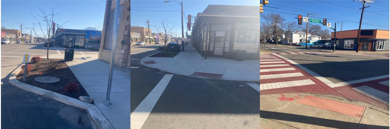
**Forest Hill Avenue: Hathaway Road to East Junction Powhite Parkway** - The project installed a five lane section with curb & gutter, sidewalks, bike lanes, closed storm sewer system, street lighting and landscaping from Powhite Parkway to Hathaway Road.
