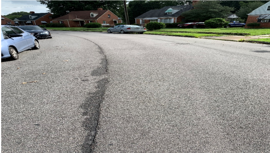
Joints separating
