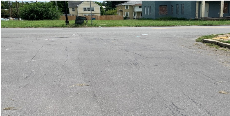
Street cracking
