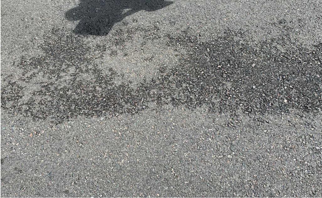
Open and segregated paving
