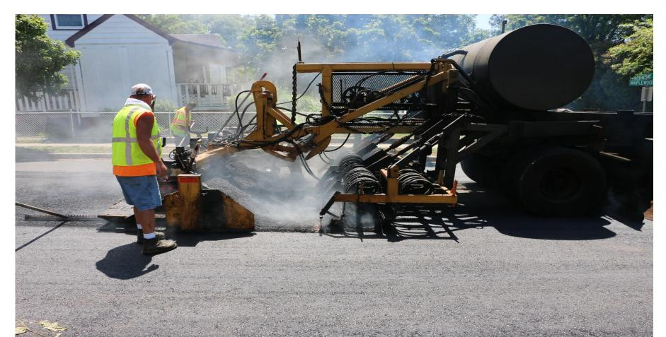
During this operation small areas at corners do not receive the prep work treatment due to the large equipment.
