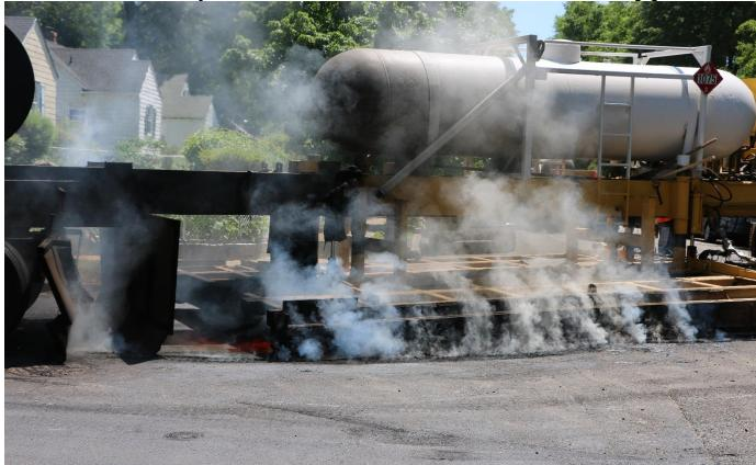
This operation is to reheat existing asphalt, scarify and re-level to smooth out the existing surface. Once this operation is complete the road surface will receive a slurry seal.
