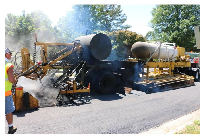
This process recycles the existing asphalt. By using this technique it prevents raising the existing utilities or changing the cross slope of existing roadways. Which speeds up the process.
