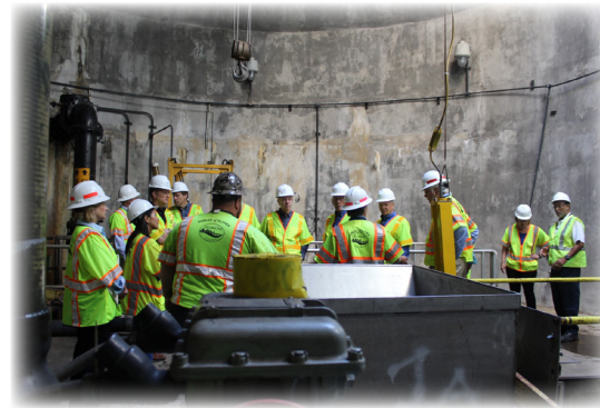
Delegation from Alexandria Renew tours combined sewer overflow system
