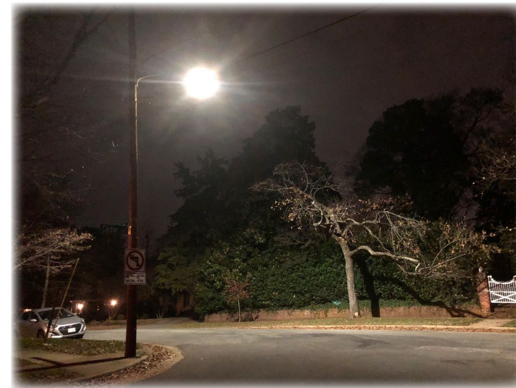
Test LED streetlight on New Kent Avenue
