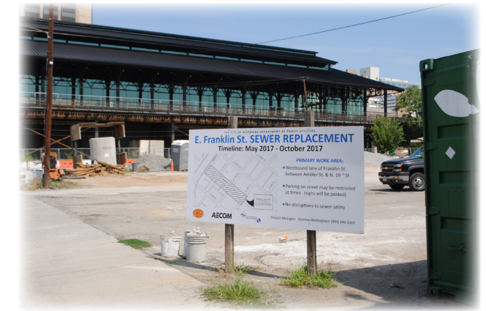
E. Franklin Street sewer replacement project
