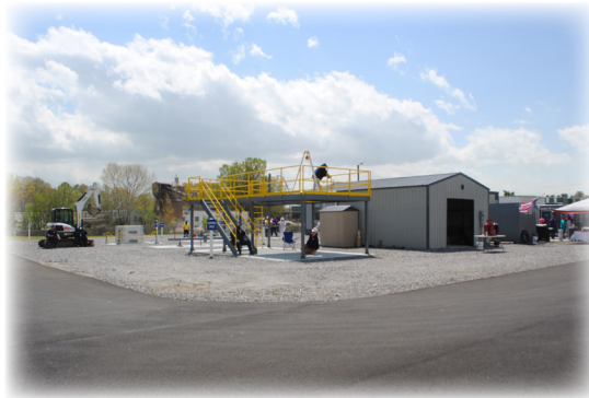
DPU Safety and Operations Training Center opened on Cardwell Road
