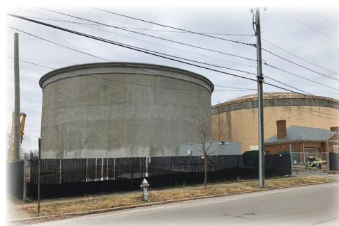
Church Hill water tank
