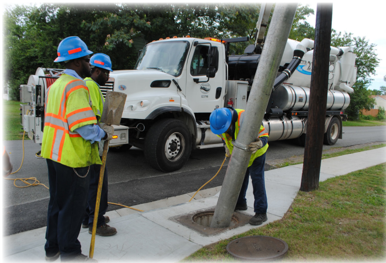
Crews cleaning debris, bottles and trash out of neighborhood storm drain
