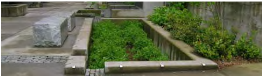
Sustainable stormwater management can be raised to the level of civic art among parks and streetscapes.
