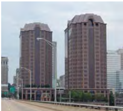
Riverfront Plaza office buildings
