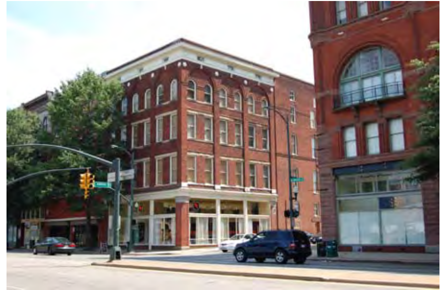
Example of Broad Street Corridor rehabilitation
