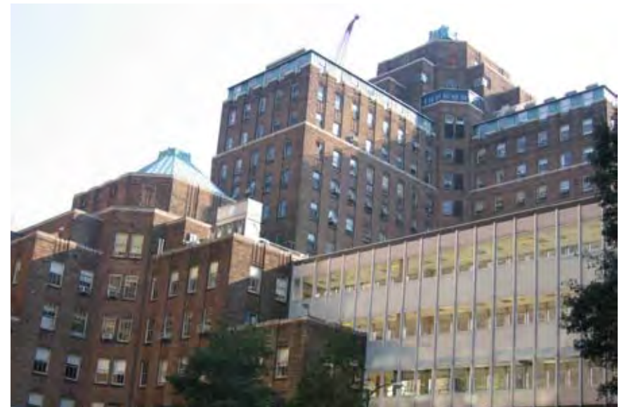
The West Hospital is owned by VCU and is planned for demolition in order to build a new School of Medicine. The University, Commonwealth and City, should be encouraged to work together to explore all options for the future of the West Hospital.
