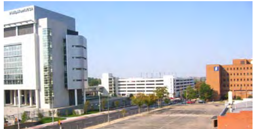
Vacant lots in the Research Park, such as this one shown above, should be developed with mixed-use buildings that front the street and respect Richmond's traditional urbanism.
