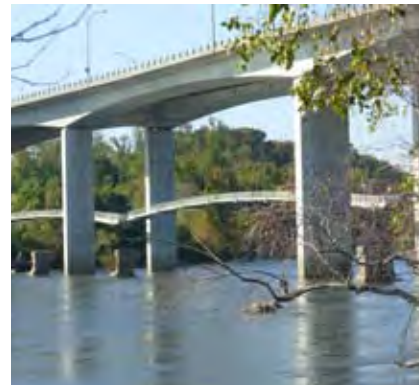
Lee Bridge with footbridge to Belle Isle
