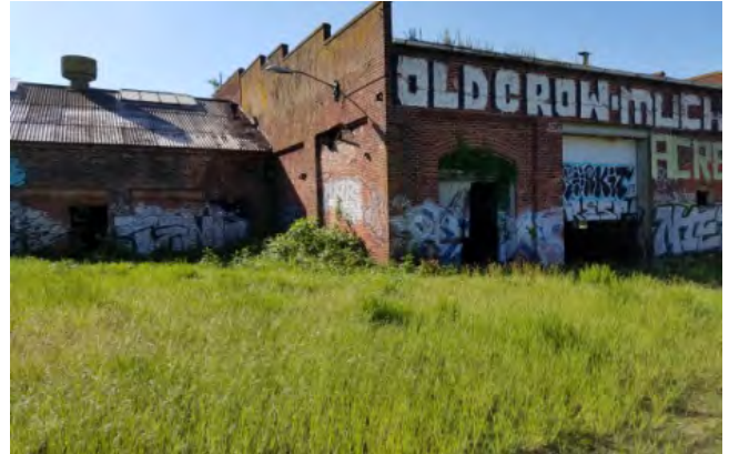
View of Building #1
