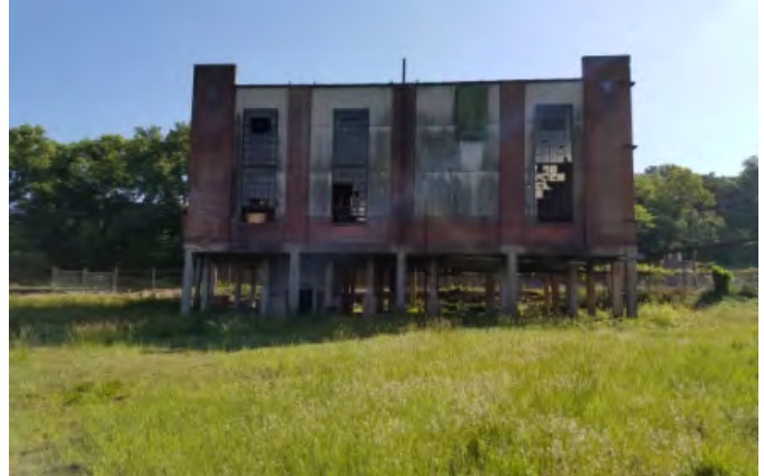
View of Building #2
