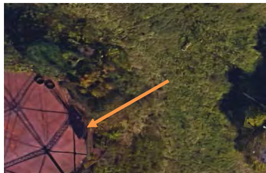
View of Shed #1
