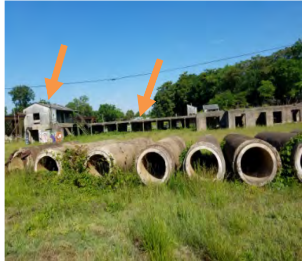
View of Building #3 & Storage Canopy
