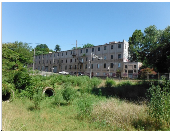
View from the north central portion of the site showing the rail line to the north of the site with the former Fiber Board Container Co. building beyond.
