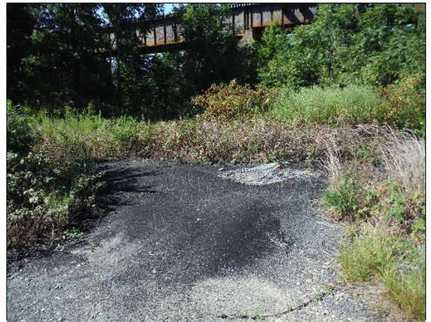
Stained soil and distressed vegetation in the southeastern corner of the site with the elevated C&O railroad and undeveloped land beyond.
