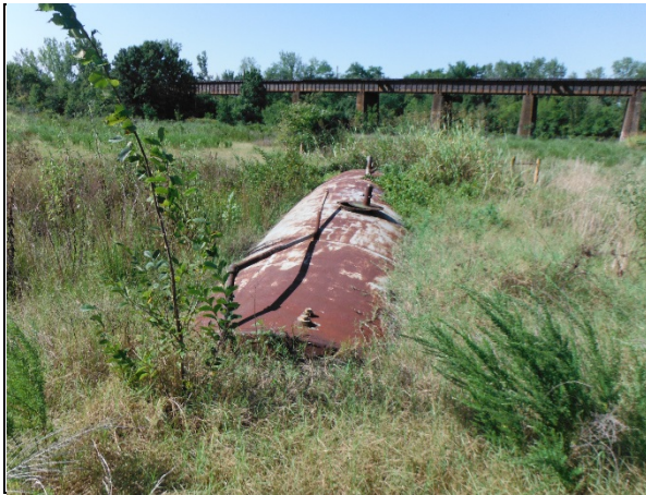
Partially buried storage tank filled with liquid and exhibiting strong hydrocarbon odors, located southeast of the engine room building.
