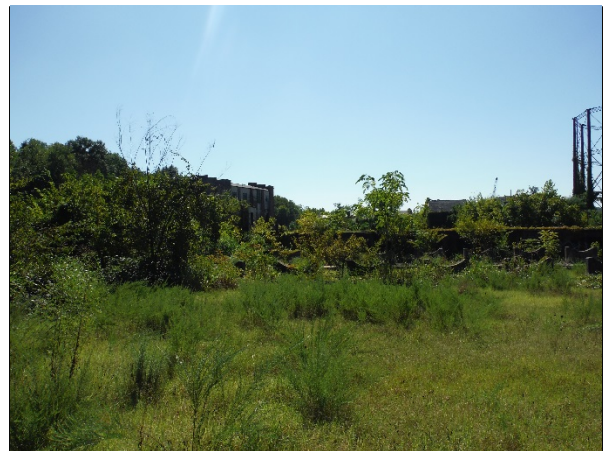
View from the northwestern corner of the site showing the former liquid gas condenser tank cradles and concrete platform.
