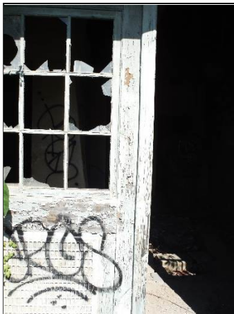
Doorway on the southern face of the engine room building showing lead paint alligator cracking.
