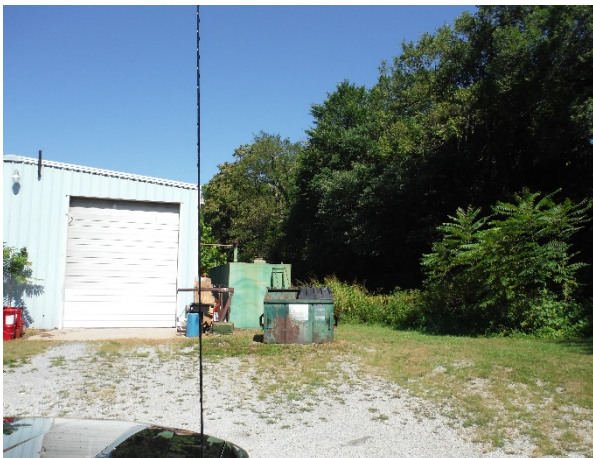
Fuel storage tanks located on the northern side of the Newton's Bus Service buildings.
