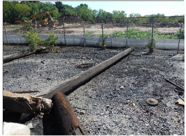
View of the southeastern corner of the site looking east, showing stained soil and construction of the Stone Brewery facility beyond. This area exhibits strong hydrocarbon odors.
