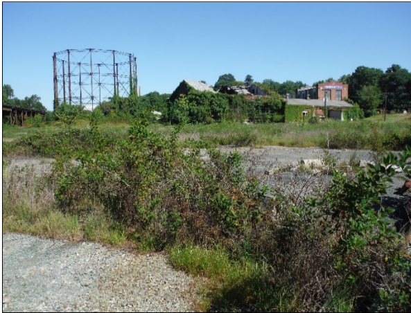
View from the southeastern corner of the site looking northwest, showing the central gasometer frame and former office, engine room and boiler room buildings.
