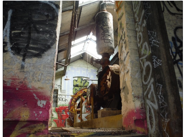
Interior of the engine room showing remnant machinery and tank structures.
