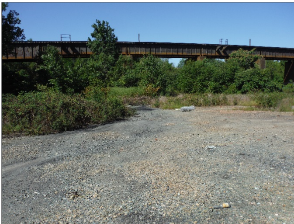
View of the southeastern portion of the site looking southwest, showing stained soil/distressed vegetation with the elevated C&O railroad and undeveloped land beyond.
