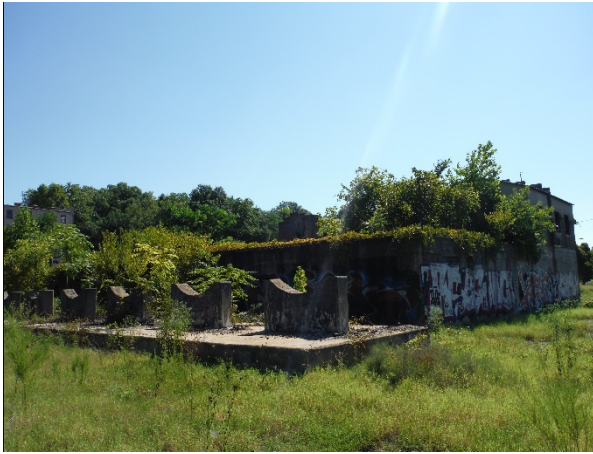
Close up view of the liquid gas condenser tank cradles, concrete platform and pump house in the northeastern portion of the site.
