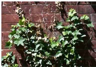
*while picturesque, climbing vines can prematurely weaken a brick wall by aiding in the deterioration of mortar joints.*
