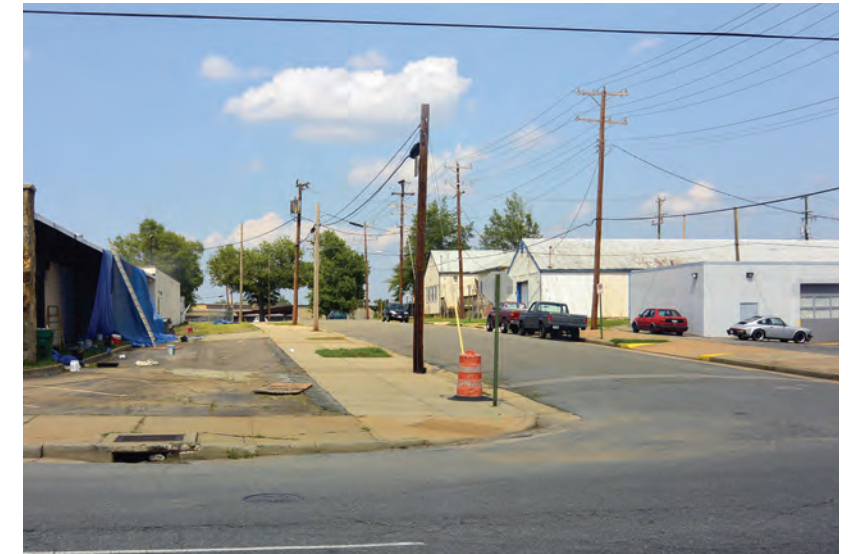
EXISTING CONDITIONS OF THE INDUSTRIAL AREA ALONG BROOK ROAD
