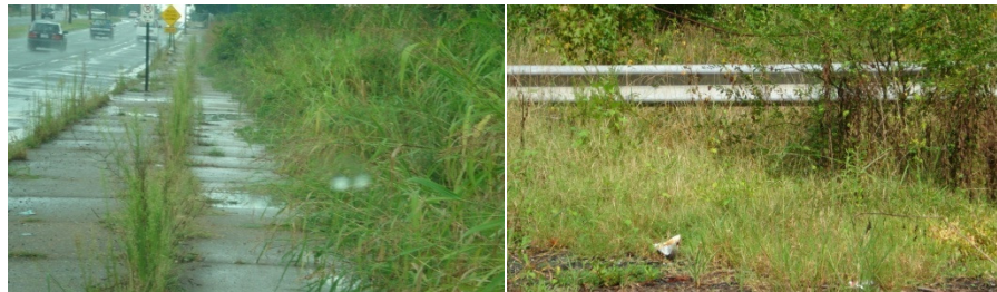
Sidewalk on Jeff Davis Highway
