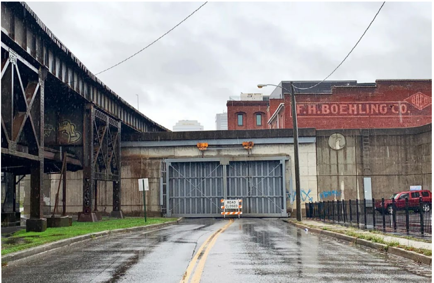
Richmond floodwall closing, WRIC
