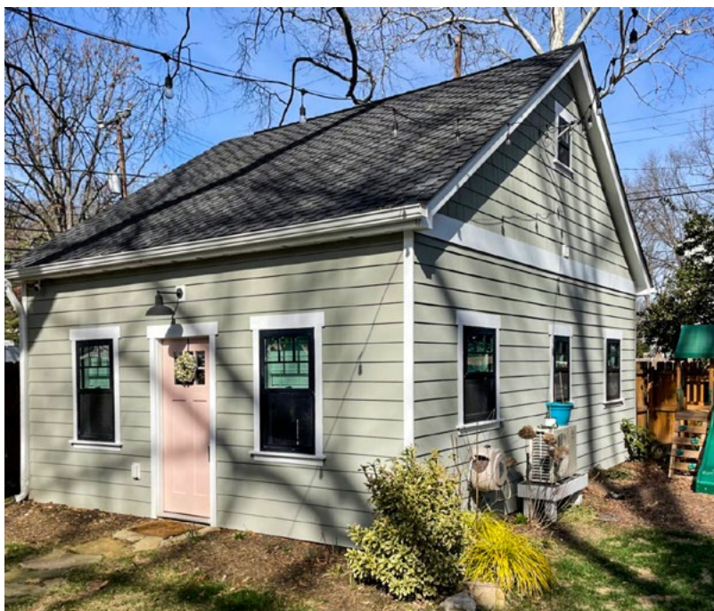
Garage to Accessory Dwelling Unit conversion, Wyatt Gordon
