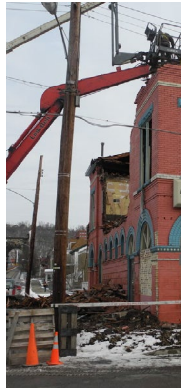
Building Demolition. CPG
