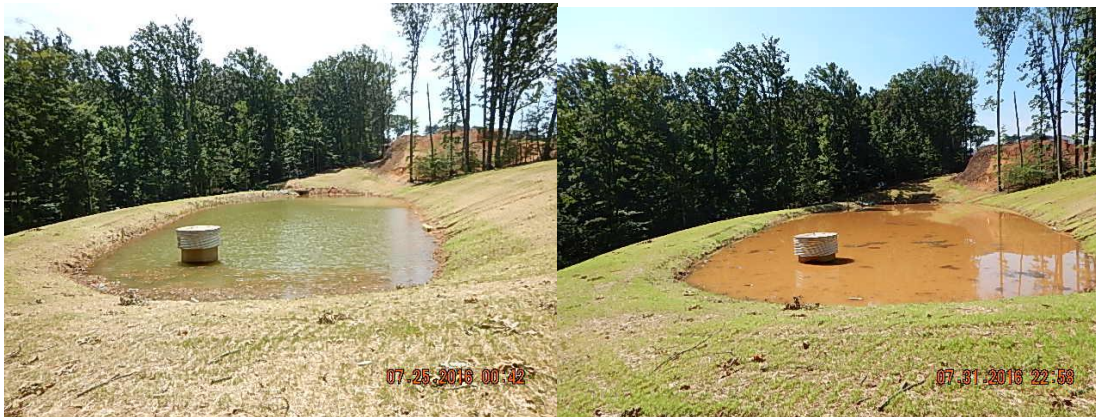
Photos of SCM at Villas at Archer Springs during construction showing vegetation growth. July 2016
