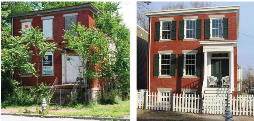
Figure 1: Rehabilitation Project before (left) and after (right)
