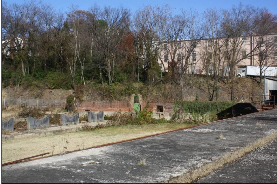
Figure 5-37. Building 3, brick wall and door, view north.
