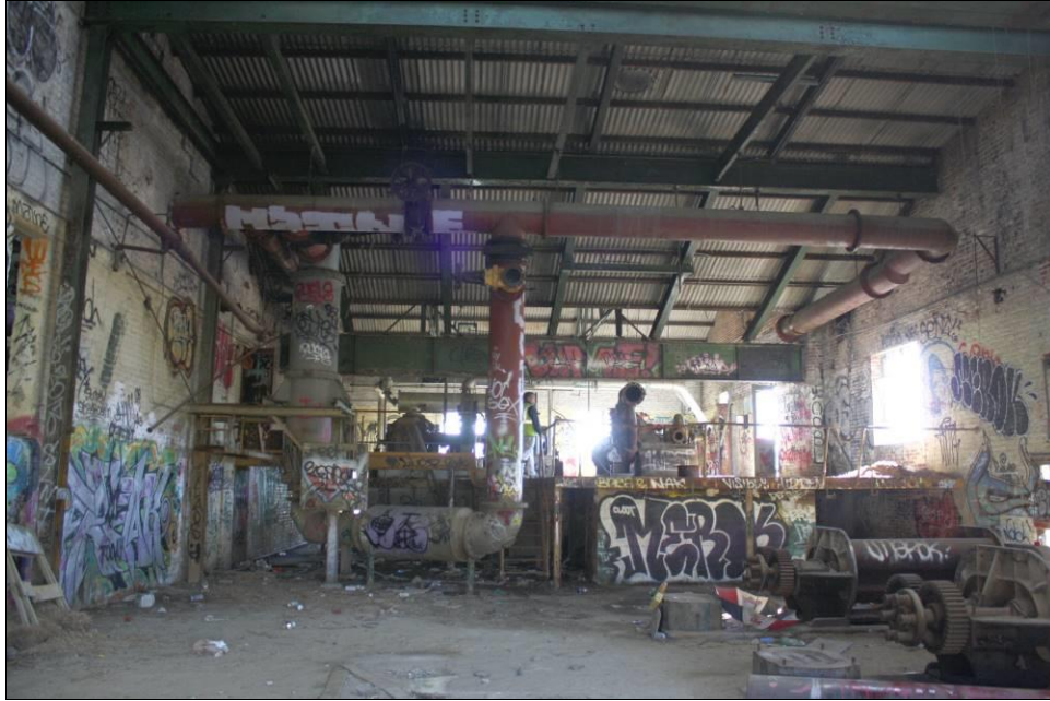
Figure 5-29. Building 2, interior of Engine Room, view southeast.
