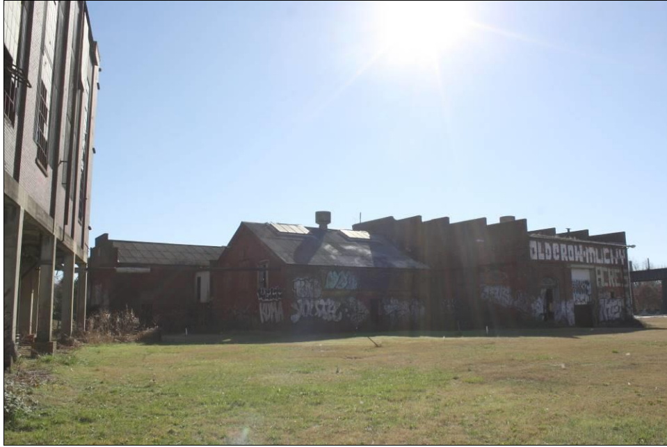
Figure 5-27. Building 2, view southeast.
