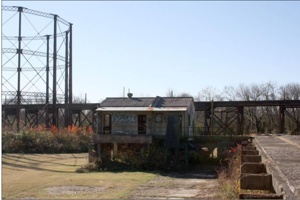
Figure 5-33. Building 3, large shed, view southwest.
