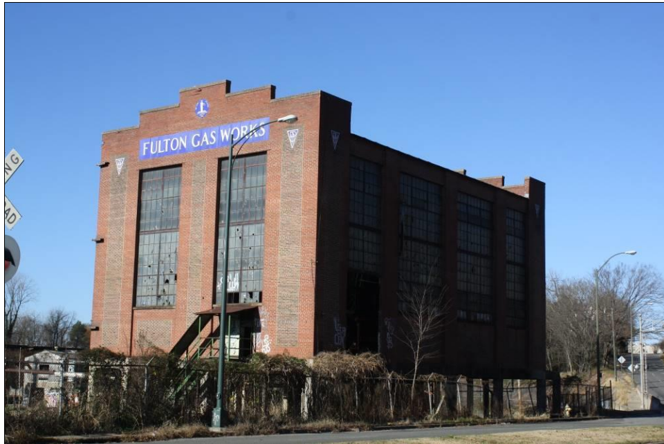
Figure 5-24. Building 1, view west from Williamsburg Avenue.
