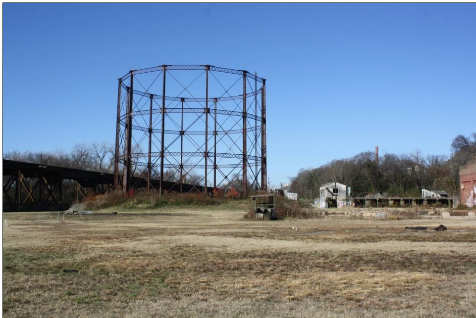
Figure 5-38. Gas Storage Tank, view northwest.
