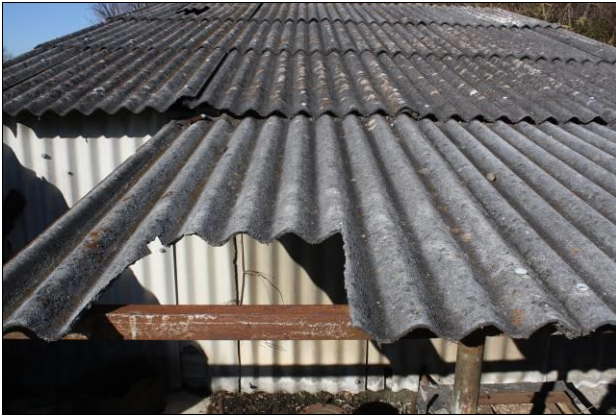
Figure 5-43. Detail of corrugated asbestos.
