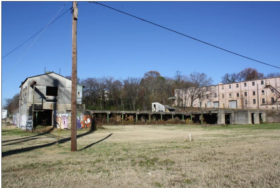
Figure 5-31. Building 3, view northwest.
