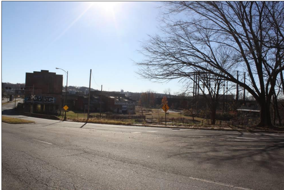
Figure 5-20. View southeast of Fulton Gas Works from Williamsburg Avenue.
