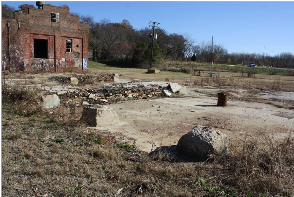
Figure 5-30. Building 2, remains of Office and Store Room, view northeast.
