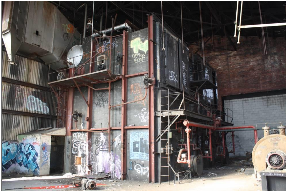
Figure 5-26. Building 1, interior view west.
