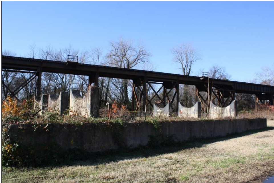
Figure 5-36. Building 3, southern Liquid Gas Condenser Tank supports, view west.
