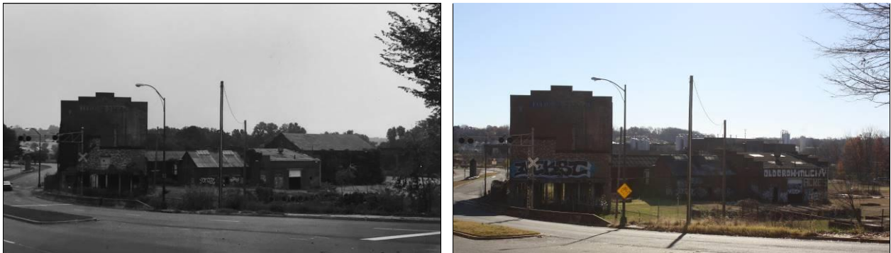
Figure 5-39. View southeast from Williamsburg Avenue towards Buildings #1 and #2, VDHR archives (left), December 2016 (right)
