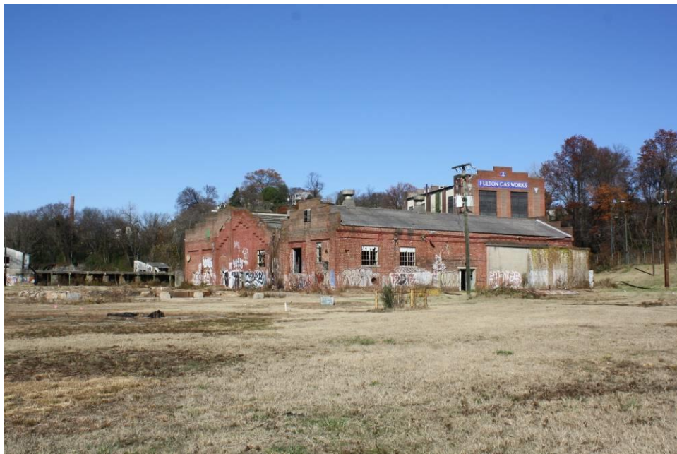
Figure 5-28. Building 2, view northwest.
