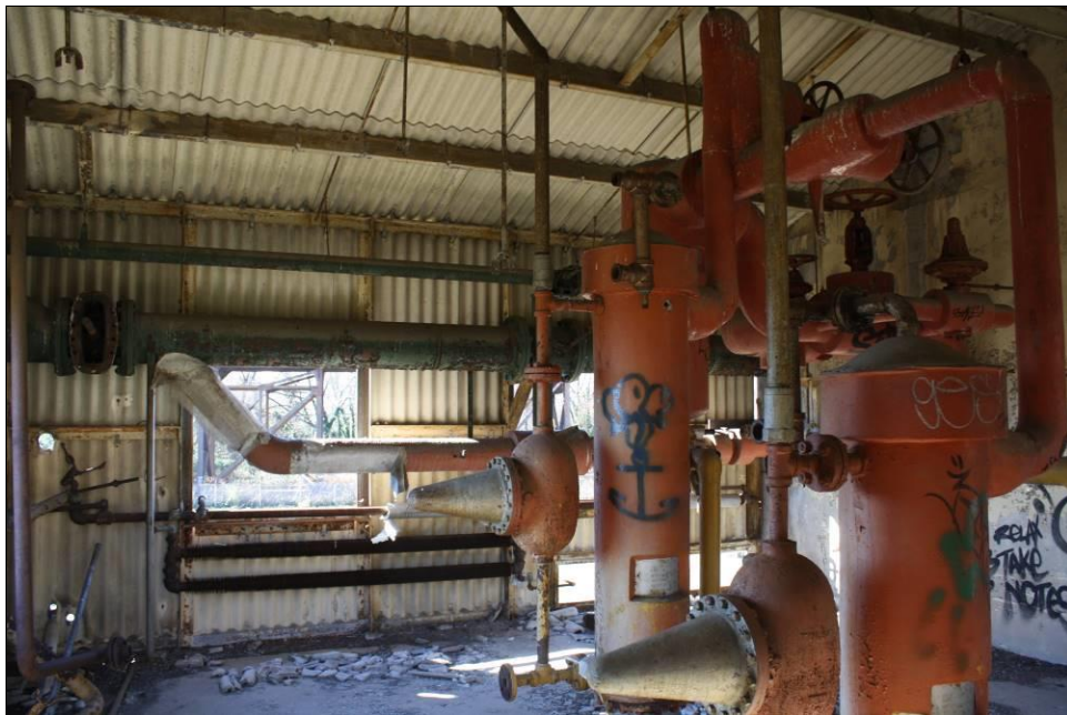
Figure 5-34. Building 3, interior of large shed, view southeast.
