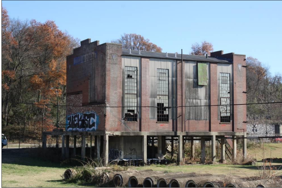
Figure 5-25. Building 1, view northeast.
