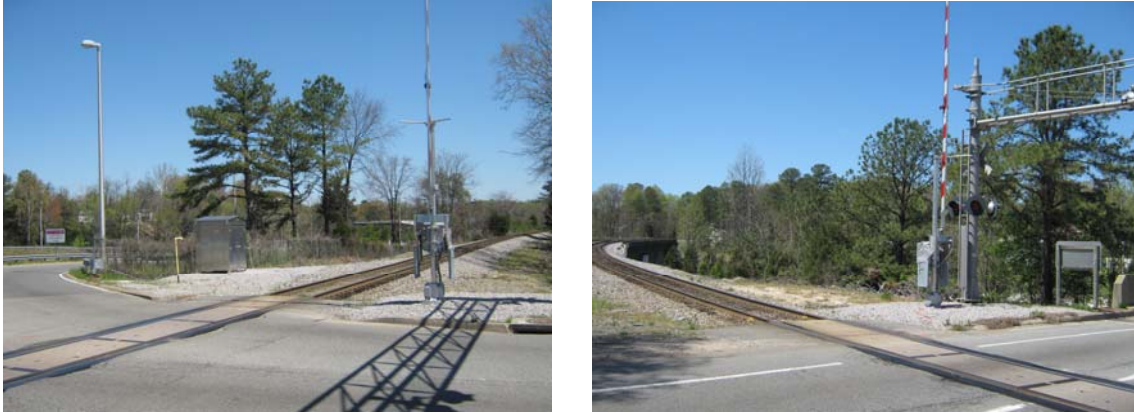
Figure 23 - At-Grade View to the North and South along the CSX Rail Tracks
