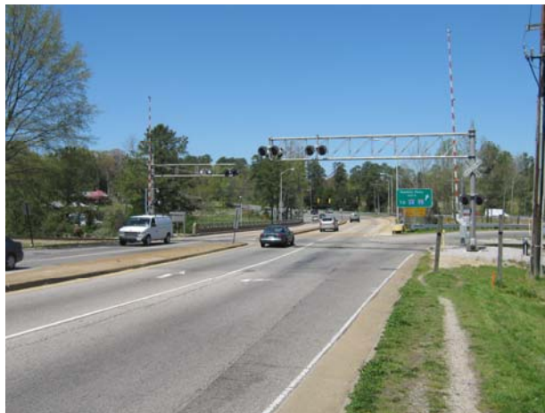
Figure 24 - Highway-Rail Crossing at Forest Hill Avenue and Powhite Parkway NB Ramps
