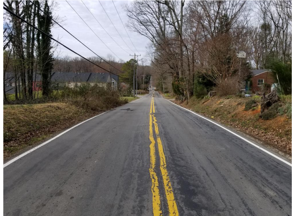
Forest Hill Avenue Facing West
