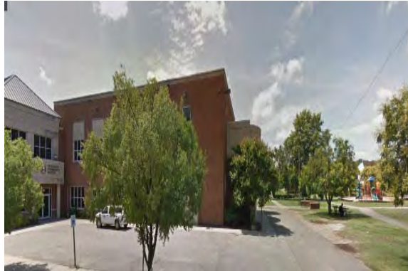
HVAC Units at Pine Camp Community Center.
