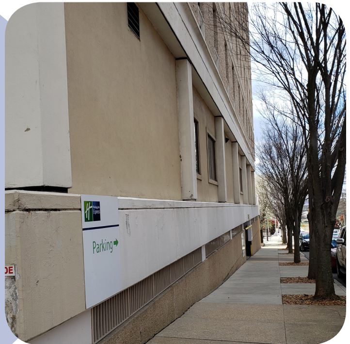
Above: a monolithic facade with little variation and no interaction with the street.
