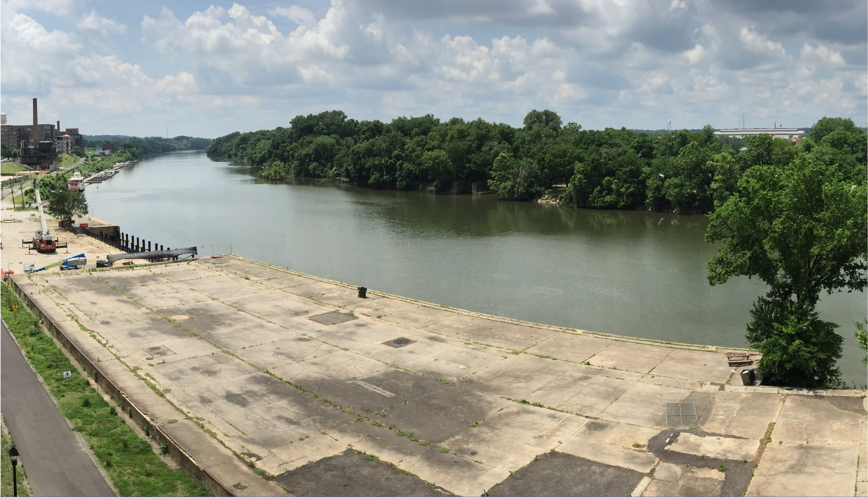
DOWNRIVER EXISTING CONDITIONS
