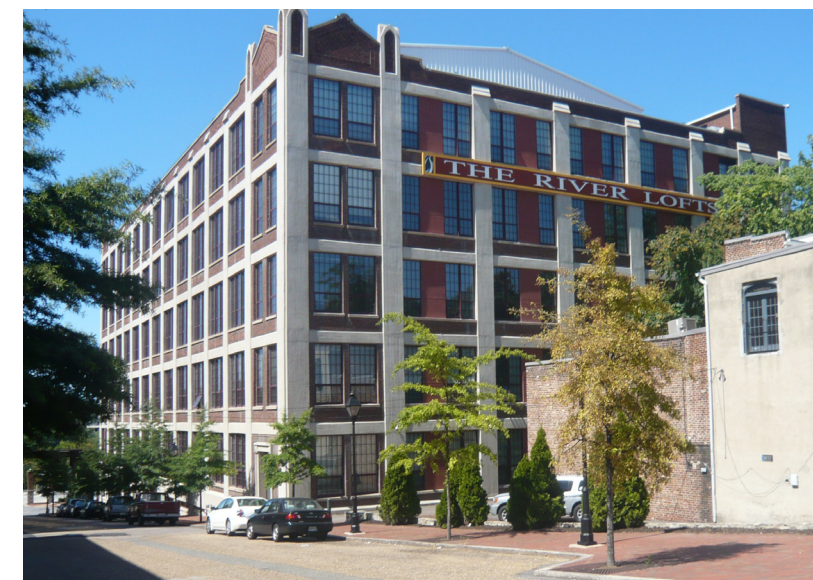
Warehouse to residential conversions in Shockoe Bottom have increased residential density and improved the jobs-housing balance.
