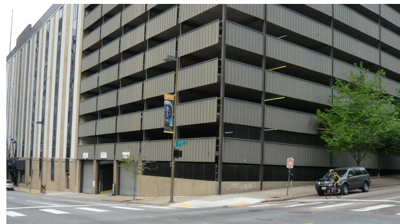
Poorly designed parking structures create gaps in active downtown streets
