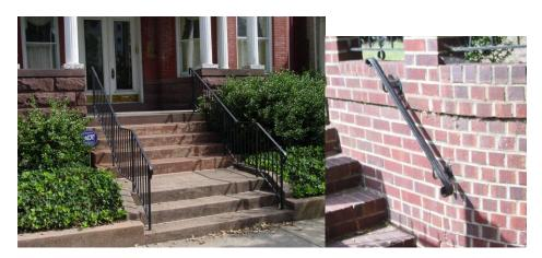
2. Staff may approve simple wooden handrails on a wooden porch or deck. Such railings must have a bottom rail, balusters, and a top rail in the manner of a Richmond Rail. Such railings may employ details such as moldings, caps, newels, and balusters that are copied literally or abstracted from the historic porch or deck to which they are attached. The following is an example of this type of railing:
