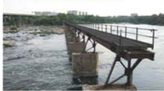
2 BROWN'S ISLAND DAM PEDESTRIAN PATH
