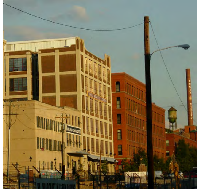
20th Century Industrial Character -- Symmetrically placed doors and windows in base, vertically and symmetrically arranged openings in the middle, and a stepped parapet at the top. Subtle variations in height, variations in color and materials to accent the organization of the elevations.
