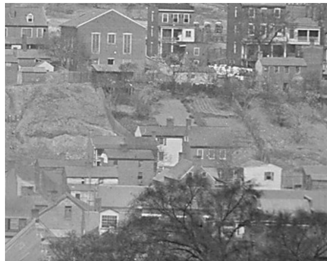
Beth Shalom Synagogue, built 1822, demolished
