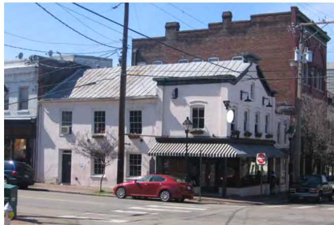
Whitlock’s Factory, built ca. 1817 1719 E. Franklin Street
