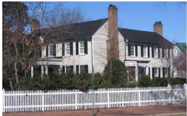
Adam Craig House, built ca. 1784 1812 E. Grace Street,
