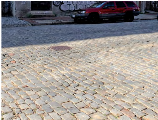
Restored cobblestone street
