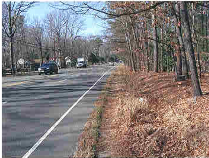
Figure 1.1 - Existing Forest Hill Avenue
